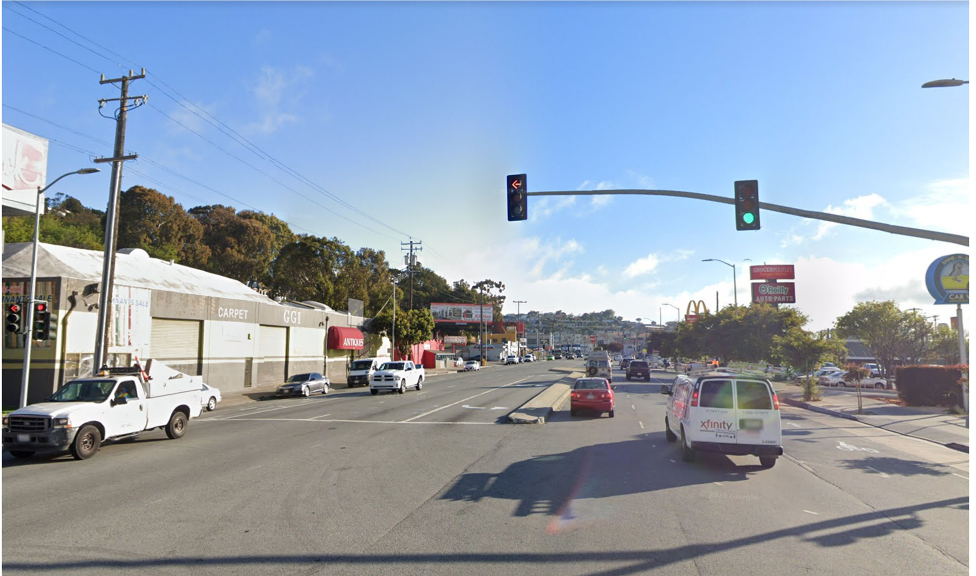
Bayshore looking north @ Lowes Signal
