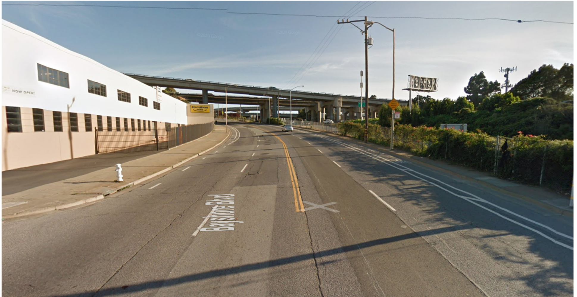
Bayshore looking south south of Industrial
