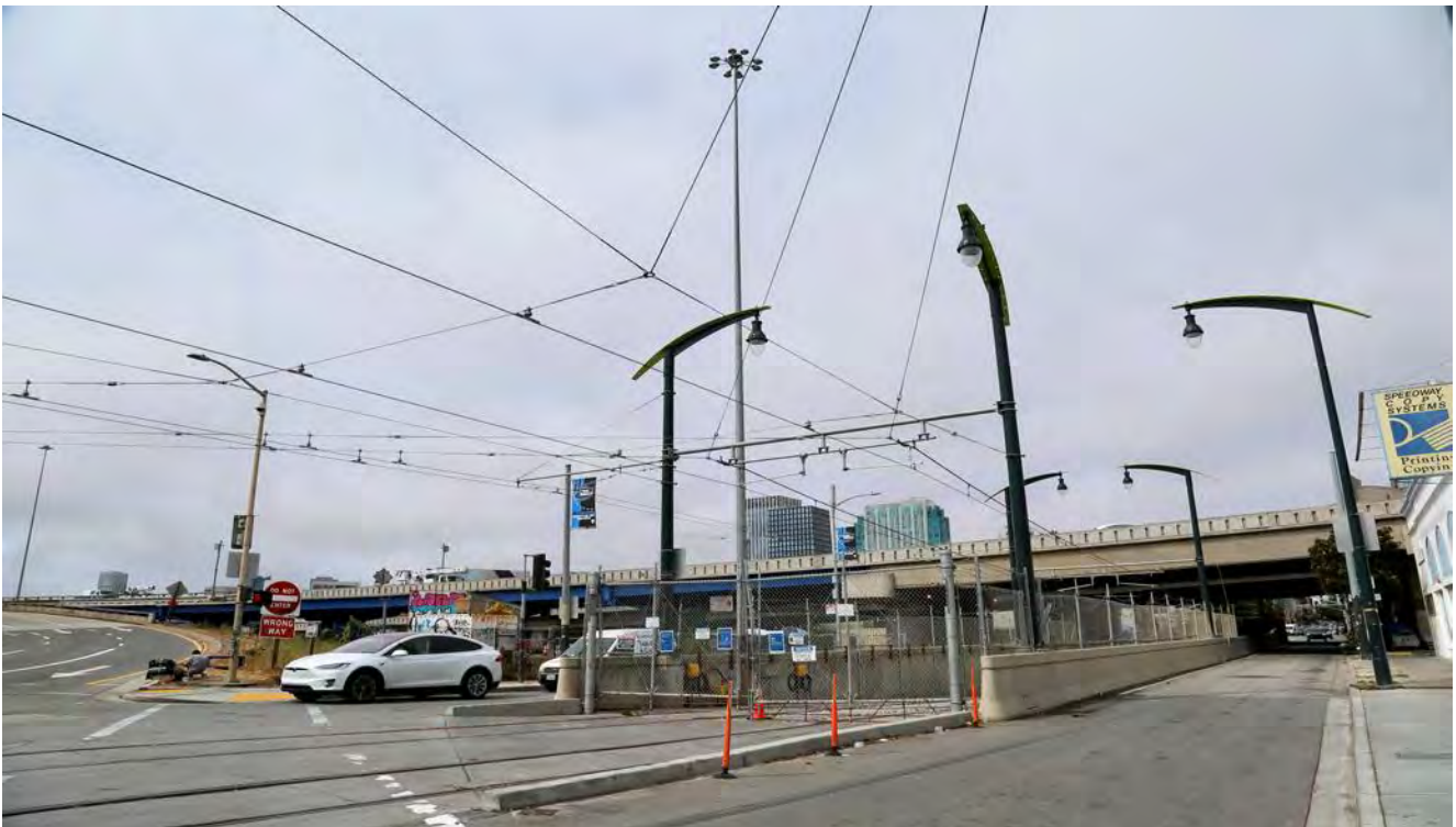
STS Portal on 4th and Bryant
