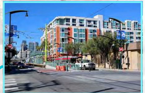
4th St. Surface Track, Systems (STS)
