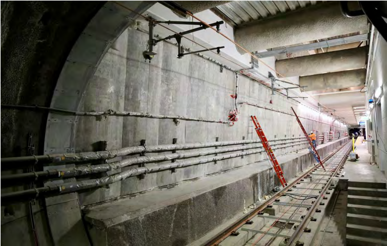
UMS view of Northbound Tunnel looking South
