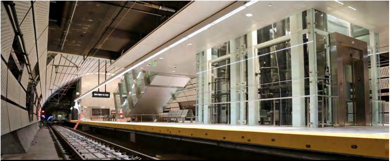
CTS Platform Level elevators and escalators
