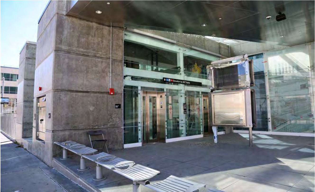
Surface level elevators and glass art
