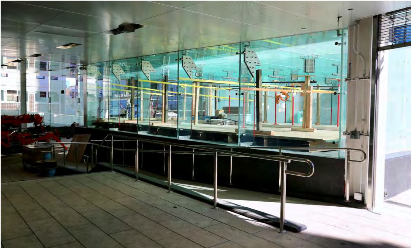
View of CTS Surface Level glass
