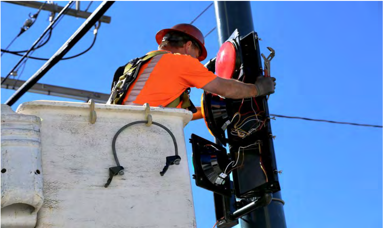
Surface traffic signal installation
