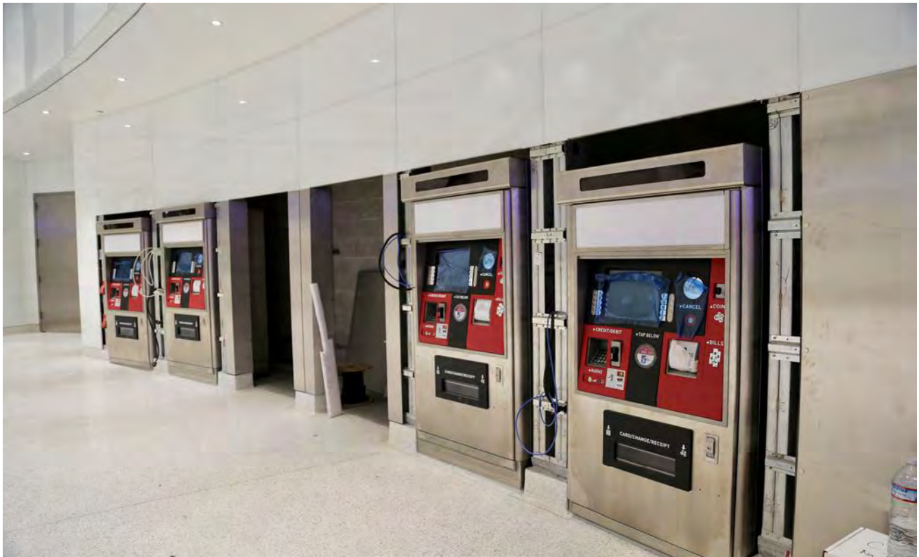
UMS Concourse Level ticket booth installation
