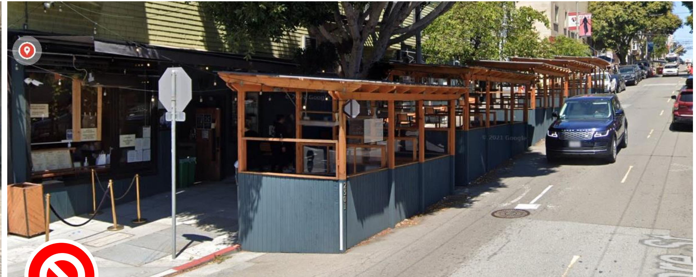
Difficult for pedestrians to see oncoming cars
