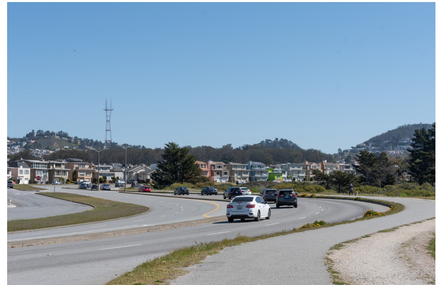
Long distances b/w crossings and gaps in signage on Lake Merced Blvd. heading eastbound towards Middlefield Dr.
