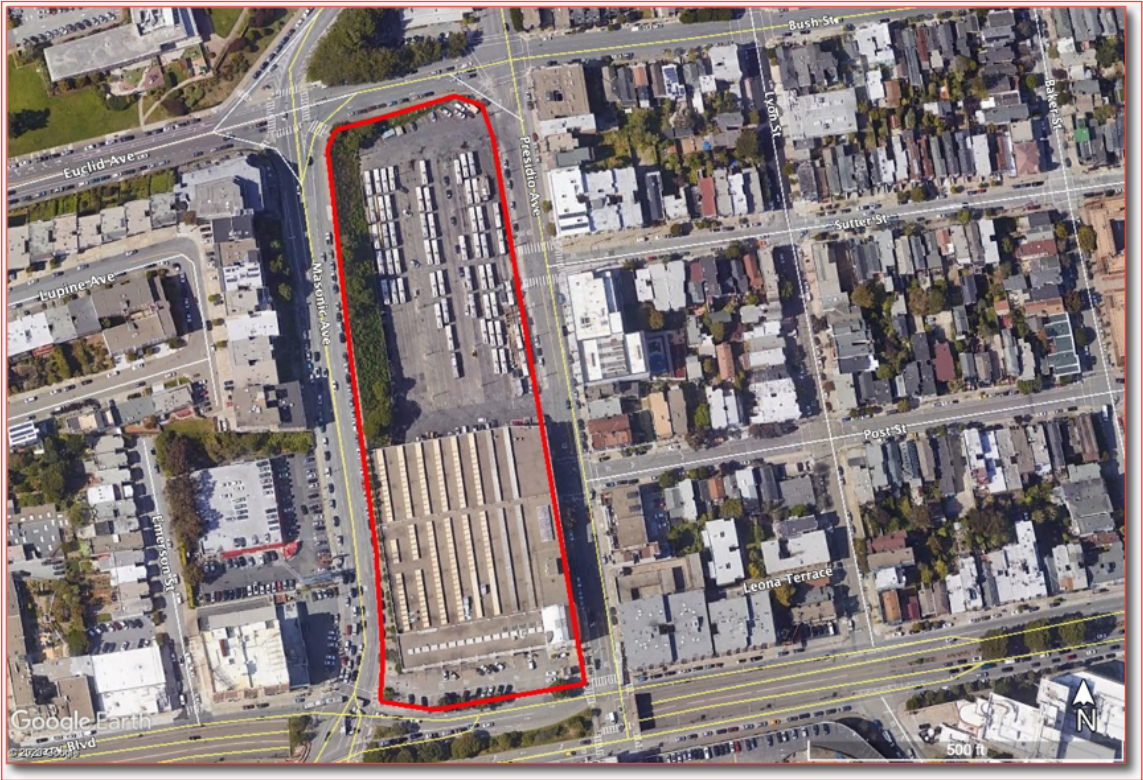
Figure 6-1. Presidio Yard - Aerial
