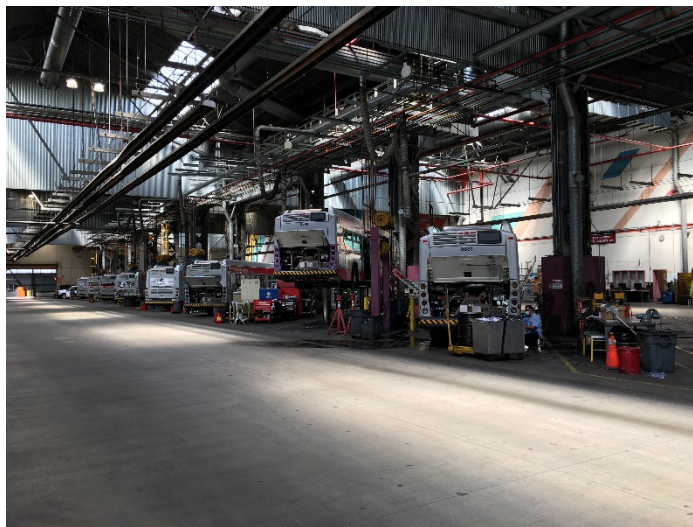
Figure 2-3. Flynn Yard - Maintenance Facility
