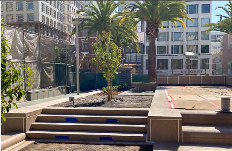
Waterproofing, terrace blocks, and landscaping are completed.
