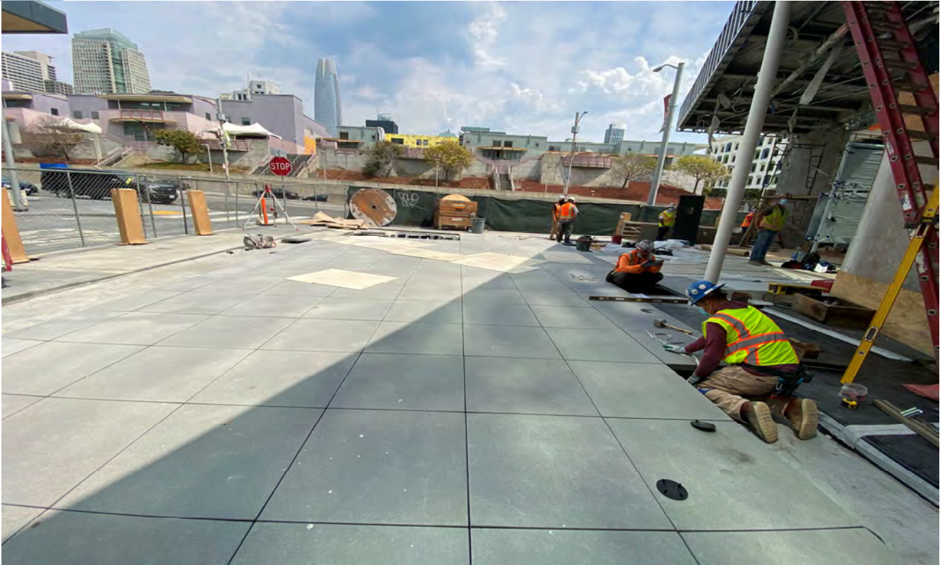
Workers installing pavers at Yerba Buena/Moscone Station surface.
