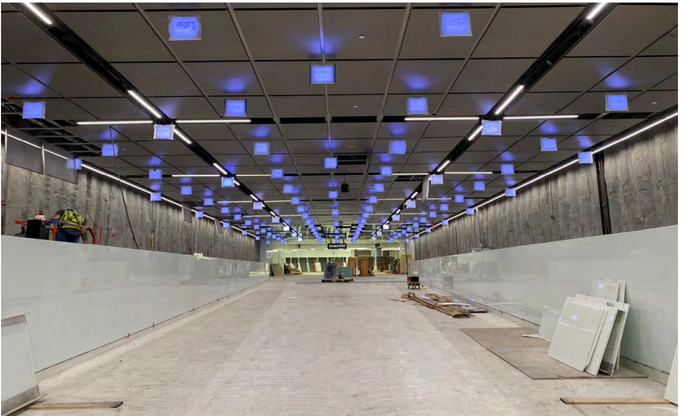
Installed Artwork Lighting at Union Square/Market Street Station concourse.
