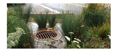
Construction work in front of City Hall is underway and with it comes an exciting addition to the project: green infrastructure. Green infrastructure is a storm water management tool that slows down and cleans stormwater preventing it from overwhleming city sewer systems.
