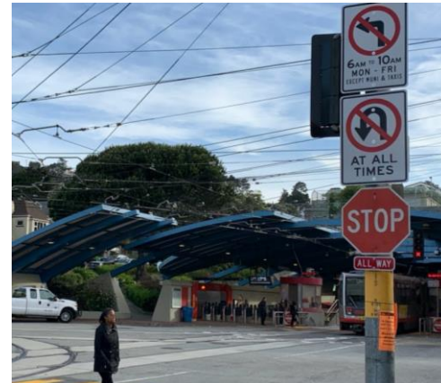
West Portal pilot
