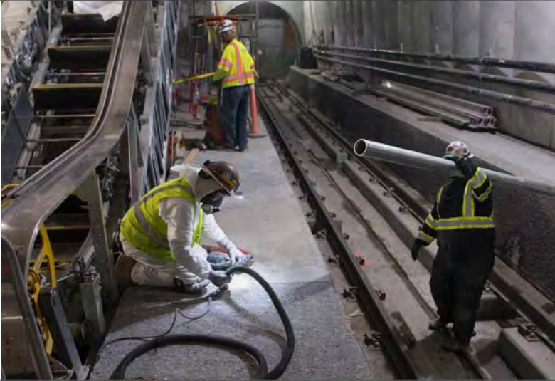
Workers prepare the surface and grind down any inconsistencies to make things level.
