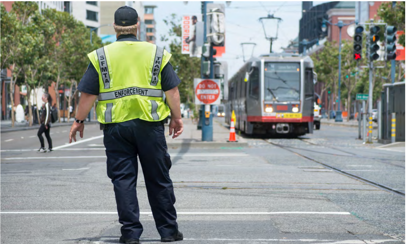
A traffic enforcement officer engages with pedestrians to maintain safety near roadway restoration work at 4th and King, as an N Judah train approaches the Caltrain platform.
