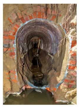
Many of the sewers being replaced are 100+ year old brick structures
