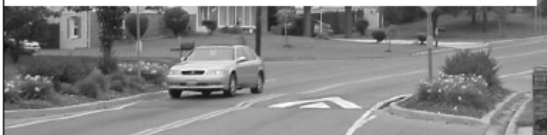
Properly designed speed bumps are an effective means of reducing traffic speeds.
