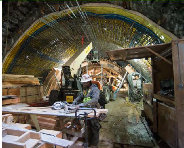
Mezzanine levels at Headhouse
