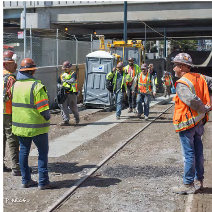
3 Crews continue installing systems from the tunnel portal to Chinatown.
