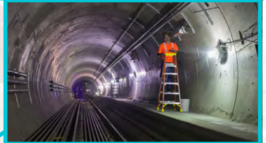
4th St. Surface Track, Systems (STS)
