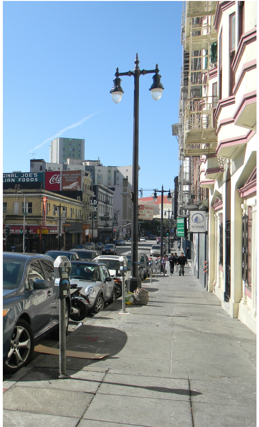
Twin Teardrop Lighting Fixtures between Turk and Eddy Streets
