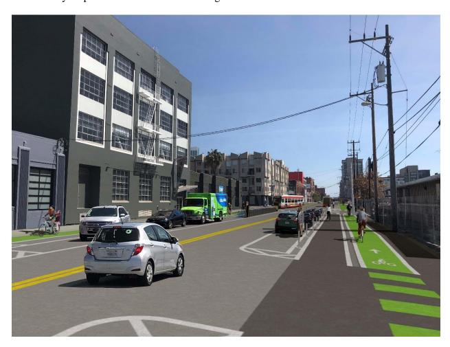
On the block between 4<sup>th</sup> Street and 5<sup>th</sup> Street, the pedestrian walkway will be further enhanced as an 11' sidewalk island, a raised concrete feature in the roadway with standard curb height that is intended for pedestrians. Similar to a transit boarding island, a sidewalk island has other
