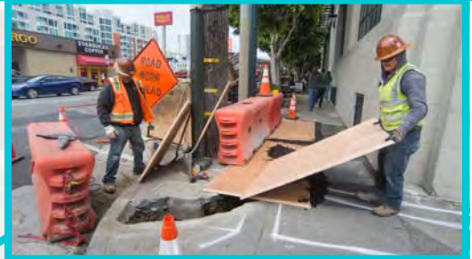
4th St. Surface Track, Systems (STS)
