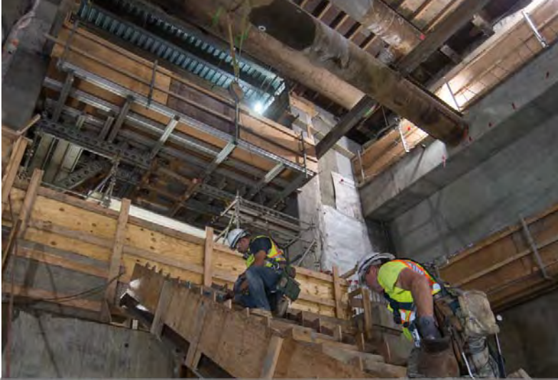
1. Workers continue installing rebar and concrete forms for stairs
