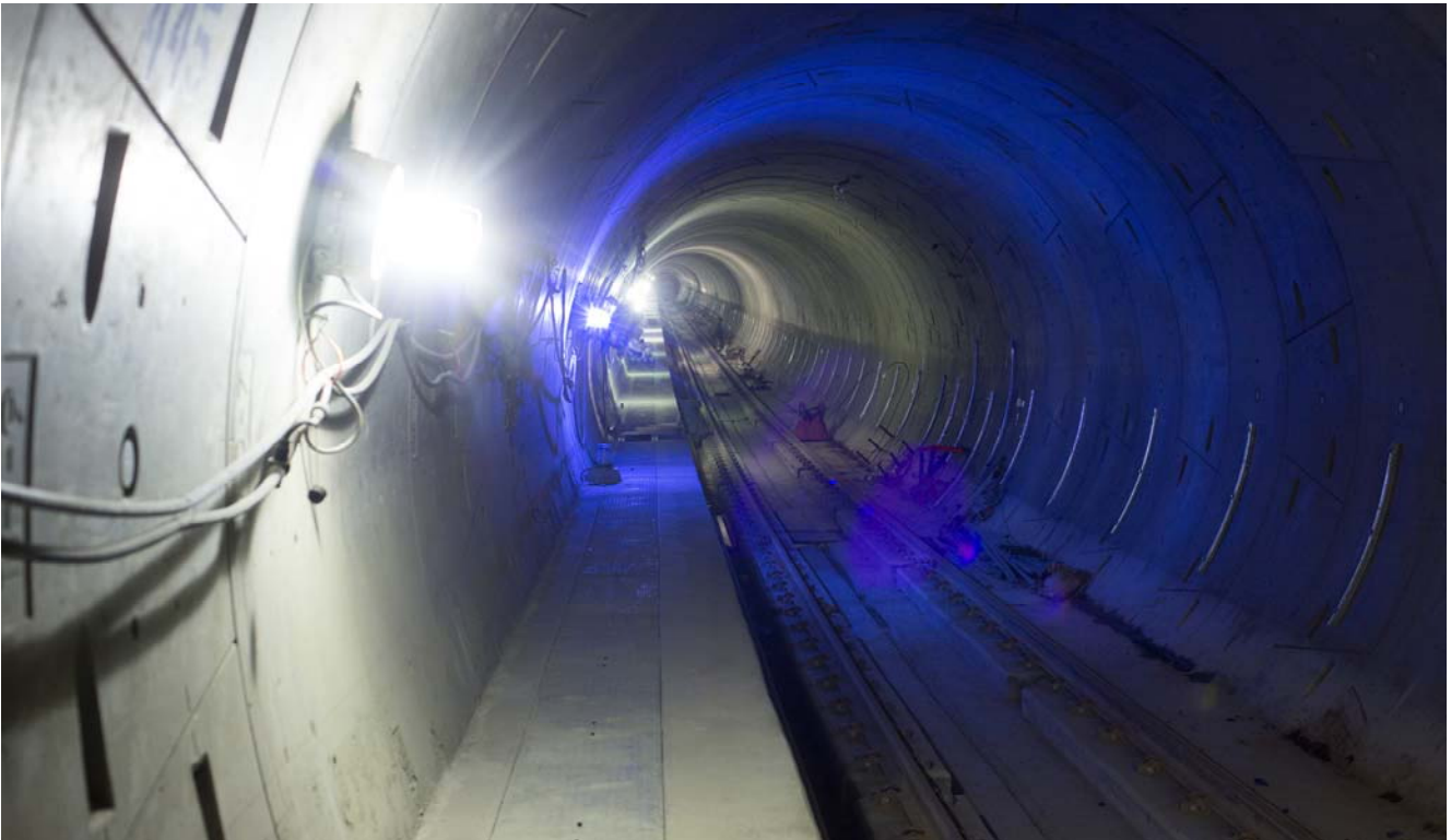
A blue light marks the location of cross-passage 5, a hallway mined out between the two tunnels for drainage, access, and safety purposes.
