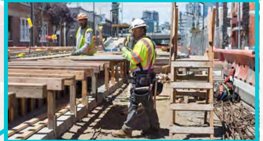
4th St. Surface Track, Systems (STS)
