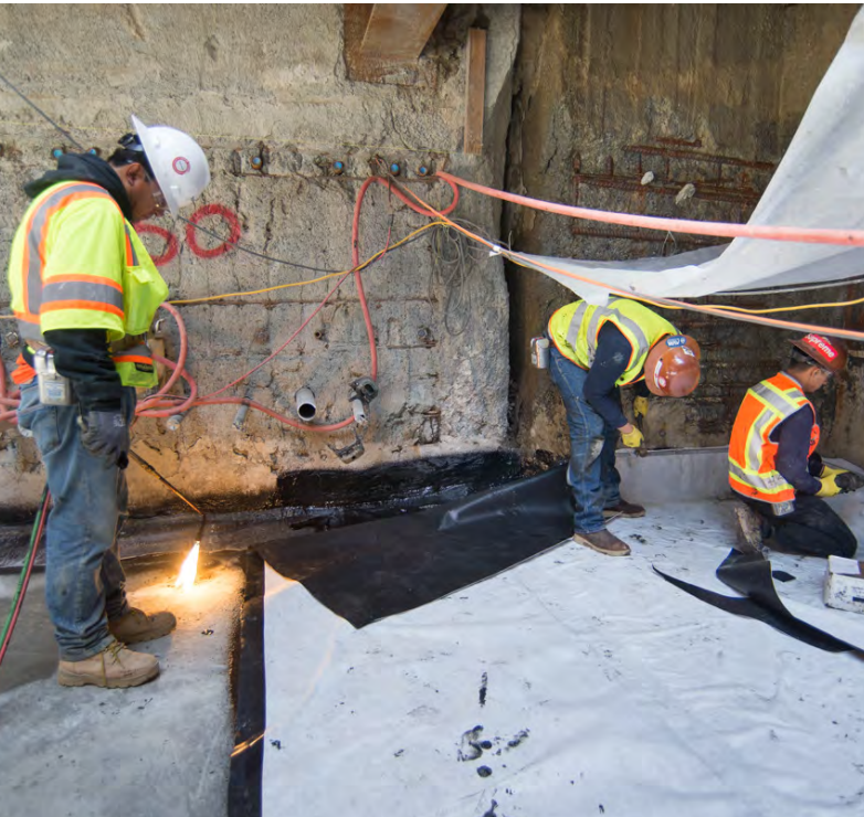
2 Site-leveling rat slab and waterproofing are installed
