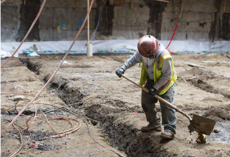
1 Trenches for grounding wires are dug and grounding wire installed
