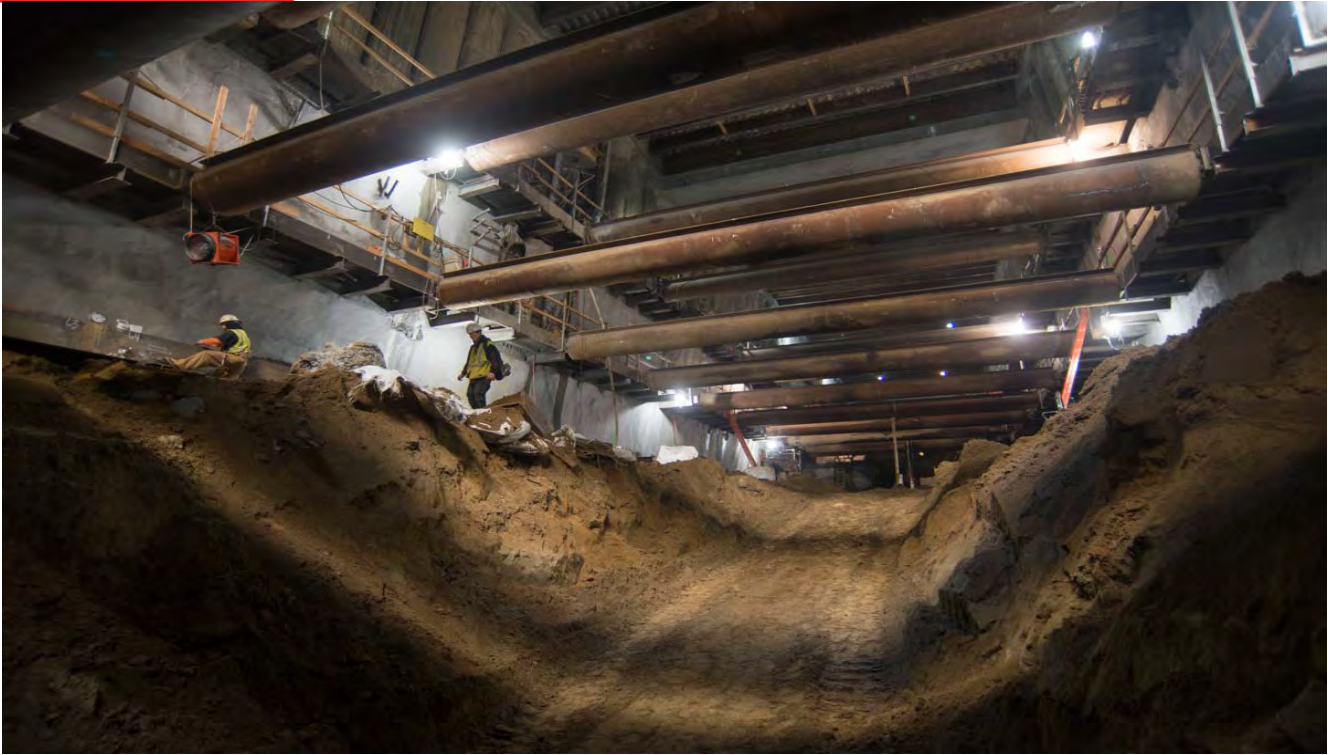
Excavation work inside the station box under Stockton Street.
