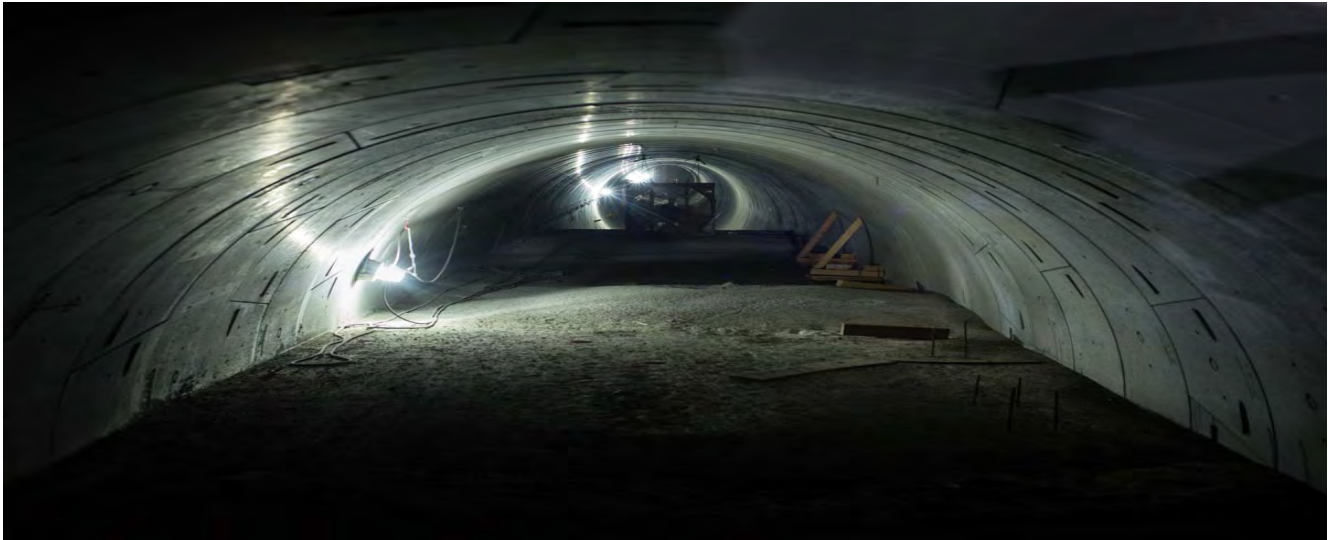
CTS Station: Crosscut view into the southwest drift excavation.
