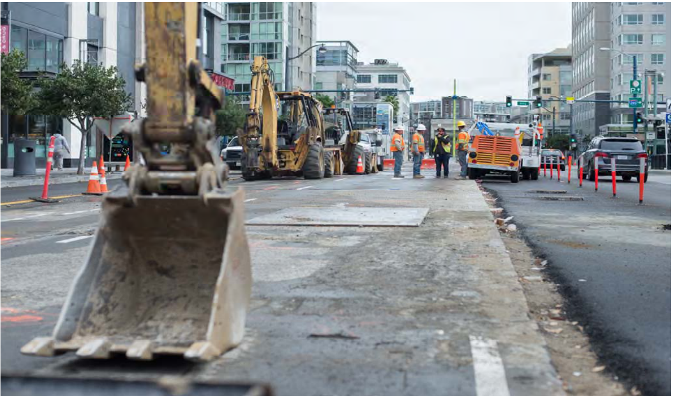
Plating over existing sewer construction.
