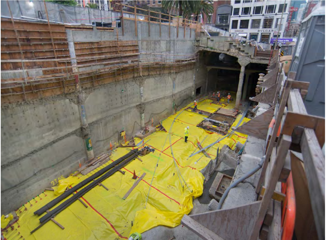
Street view of the UMS Garage waterproofing work.
