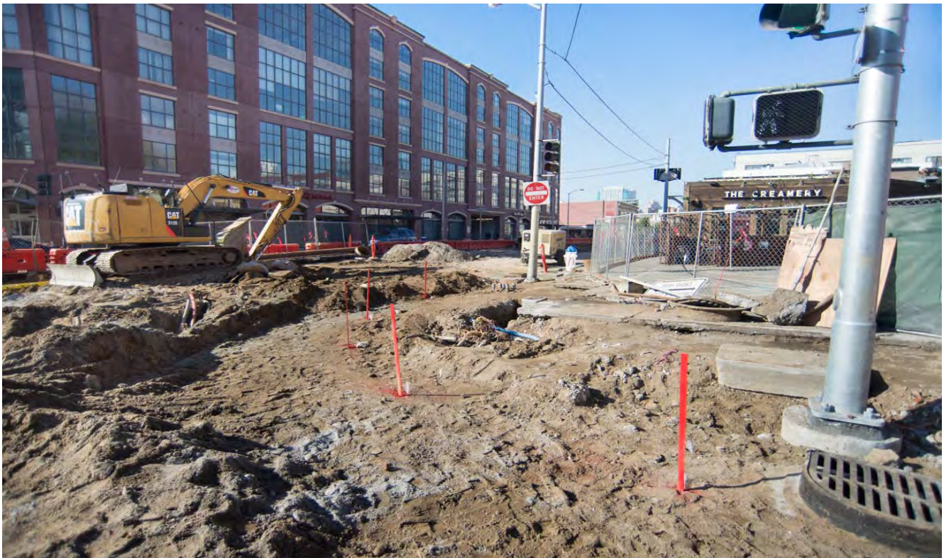
Subgrade preparation for pavement renovation at 4th and Townsend.
