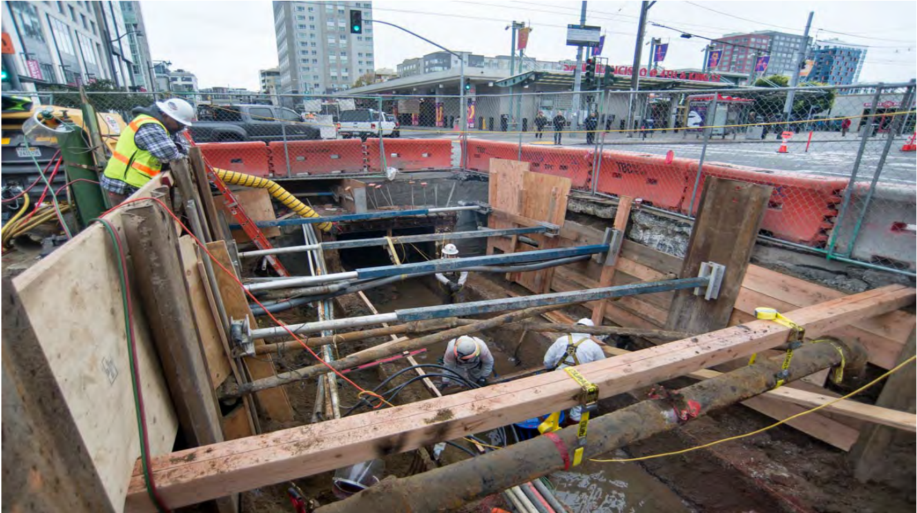
78" sewer improvement at 4th Street, north of Townsend.
