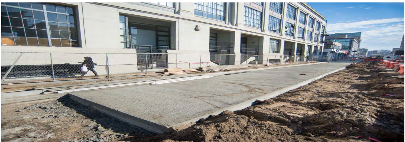
Street restoration improvements at 4th Street and Bluxome
