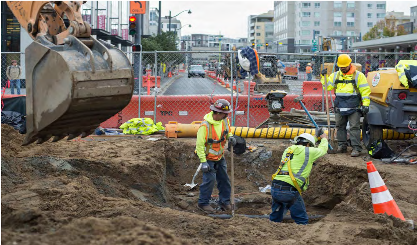
Excavation for 78" sewer offset manhole at 4th and Townsend.
