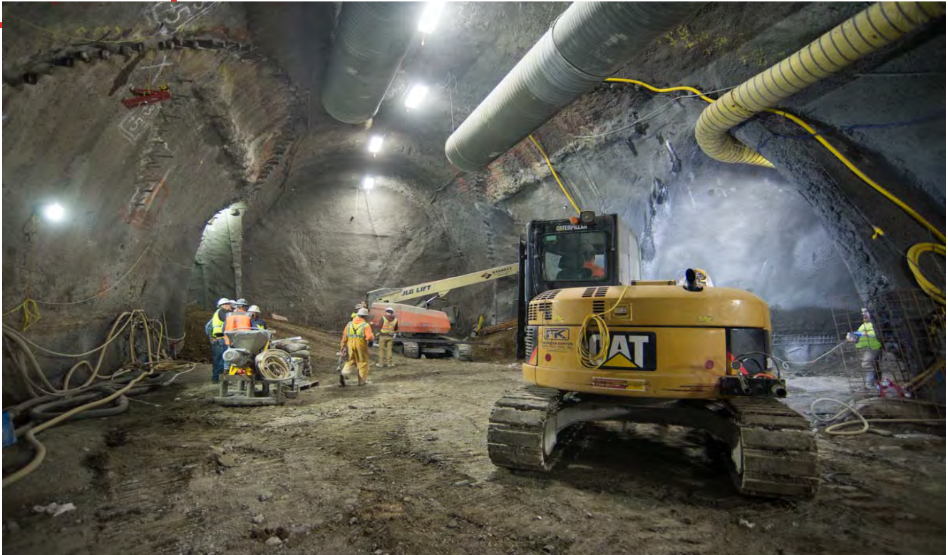
With the first phase of drilling and soil grouting complete, work to excavate the side drifts of the south platform cavern area has begun.
