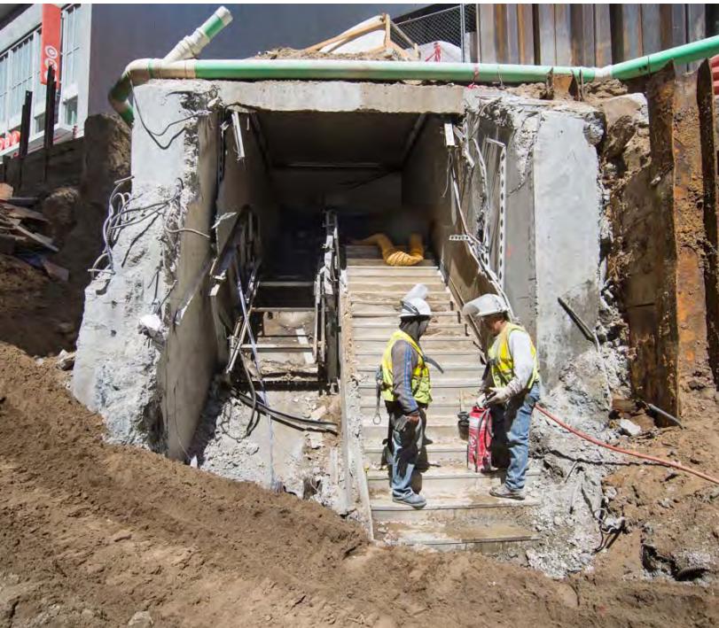
2 Redundant elements of the Powell Station entrance are removed where needed
