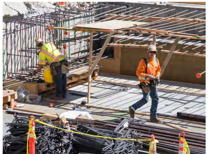
A carpenter works to construct concrete forms used to build the station roof slab.
