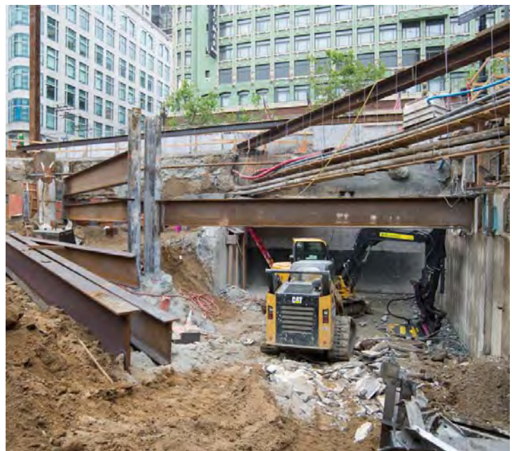
3 Workers begin installing steel beams to support the future roof structure
