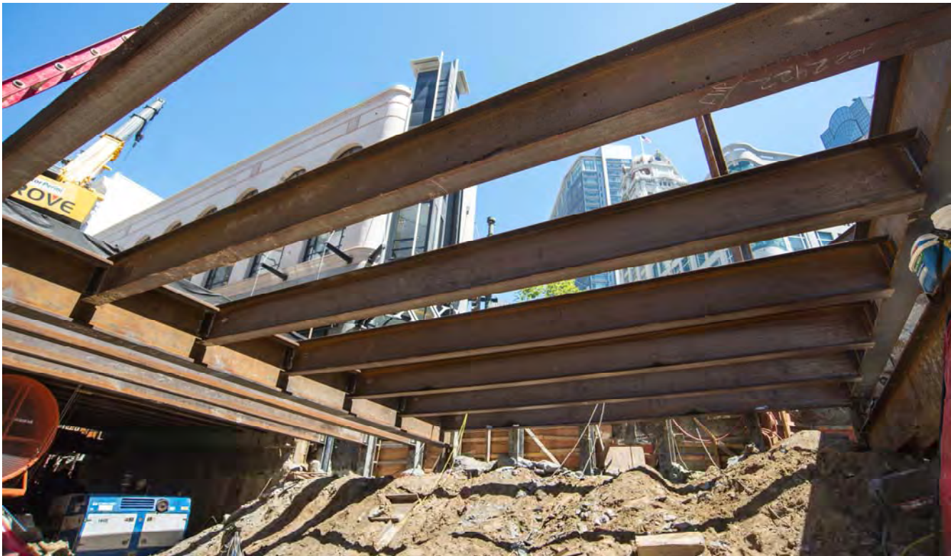
Excavation and internal structural elements will continue underneath the finished roof.
