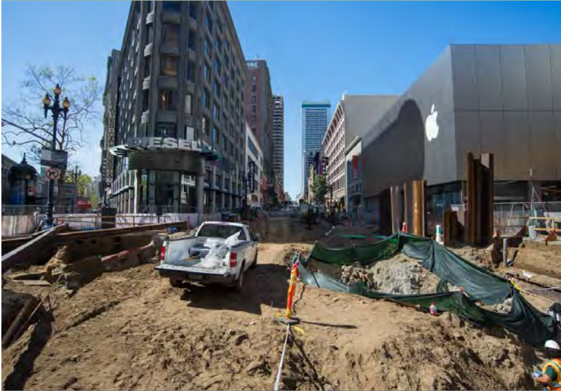
1 Pavement is removed, and ground-reinforcing steel sheet piles are installed
