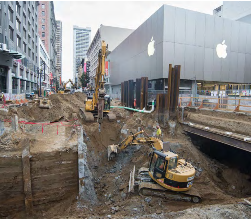
2 Soil is excavated, revealing former Ellis entrance to Powell BART/Muni station
