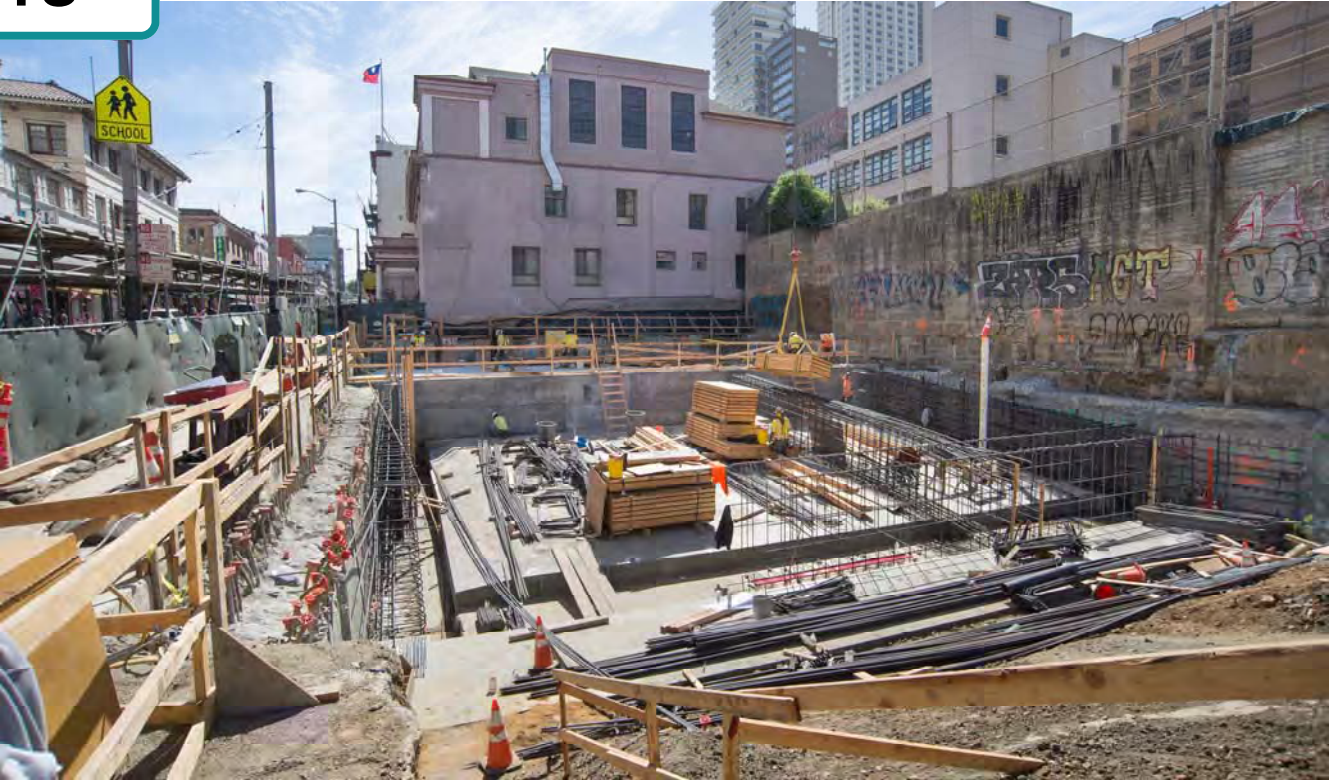
A temporary “rat slab” is being constructed as the bottom of a form which will be used to build the future roof slab of the station.
