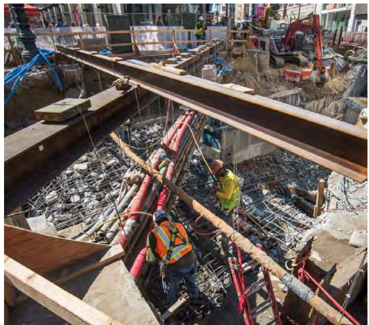
3 Workers suspend active utilities from I-beams and demolish entrance
