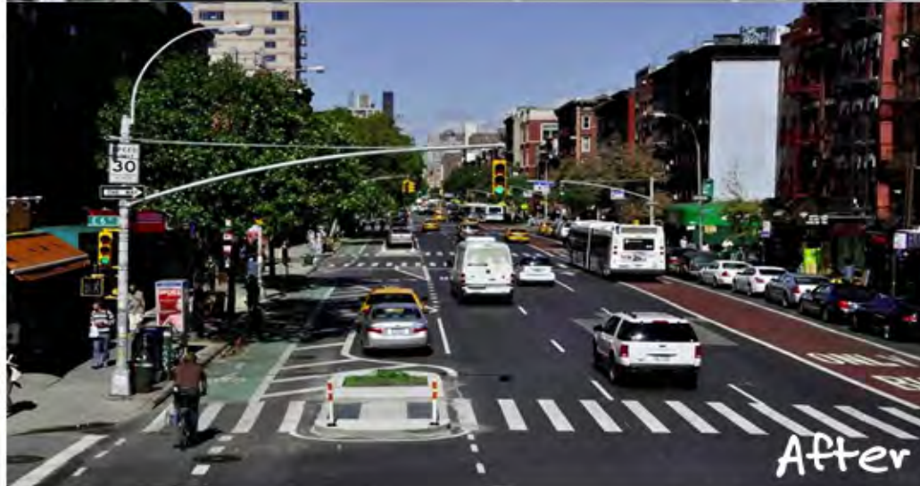
First Avenue Improvements, New York City
