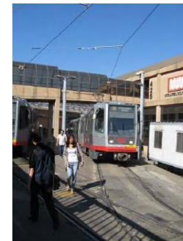
J/K Walkway Improvements
