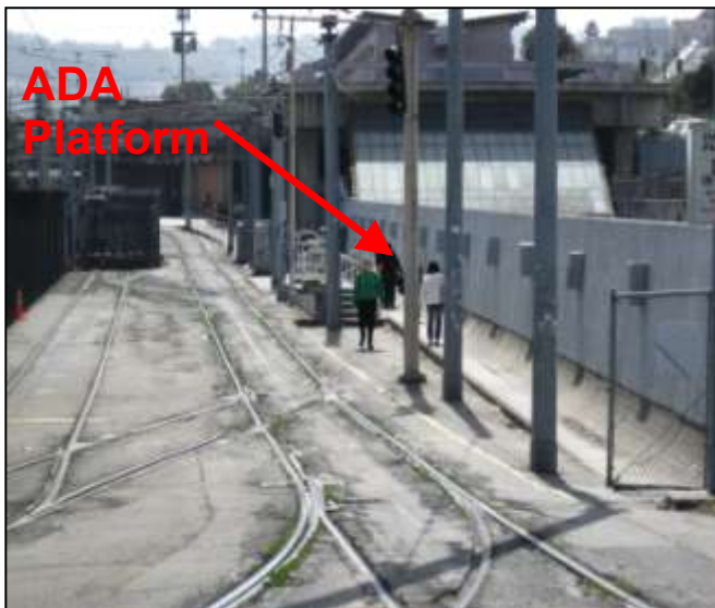
Figure 7: J/K Line ADA Platform Picture of narrow ADA Platform adjacent to LRV tracks.
