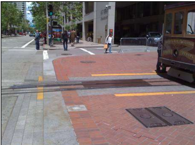
Figure 31: Example Treatment for Rail Tracks across a Curb at the Cable Car Terminus on California Street at Drum Street in Downtown San Francisco (Source: Ped and Bike Project ) Pedestrian Zone delineated with brick, a different paving material.
