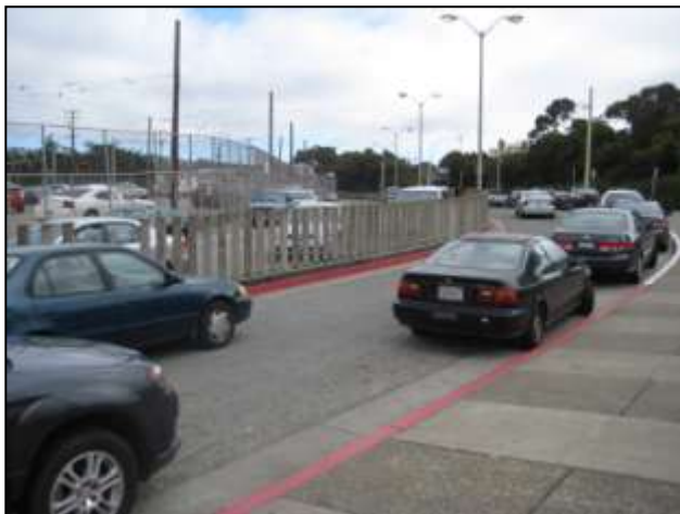
Figure 34: Lack of ADA curb ramp from kiss-and-ride to South Geneva Transit Plaza Photograph showing no curb ramps and cars parked along the red curb at the kiss-and-ride.
