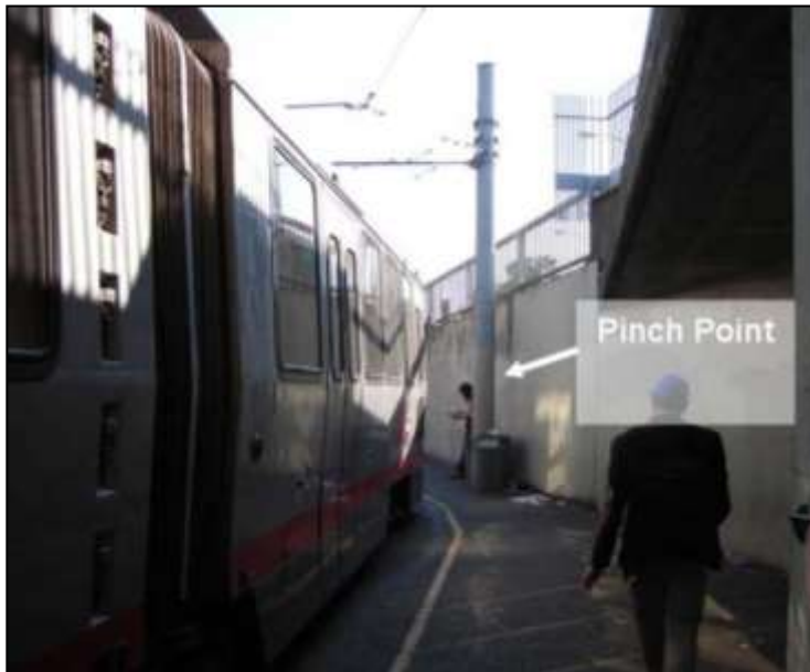
Figure 12: Pinch Point Created by Traction Power Pole. Picture shows narrow space between the traction power pole and LRV swing out area.
