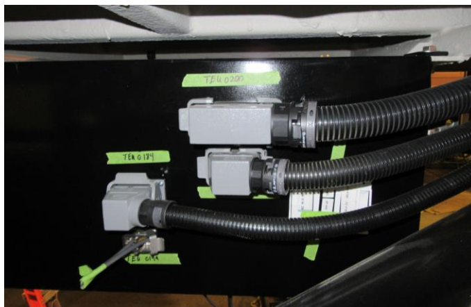
Figure 15 – Connectorized LVPS Enclosure Electrical Connections
