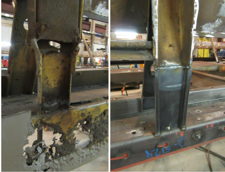
Figure 23 – Side Wall Post Bottoms Replaced
