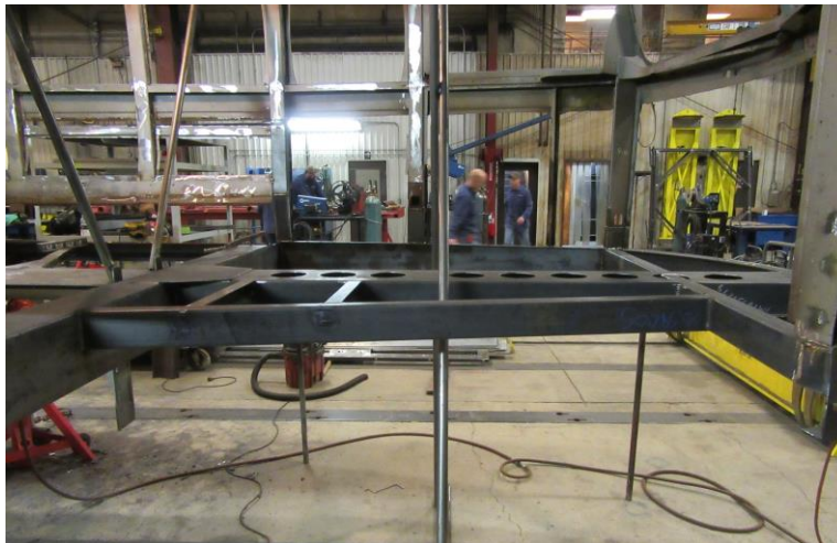
Figure 24 – Front End Replaced
