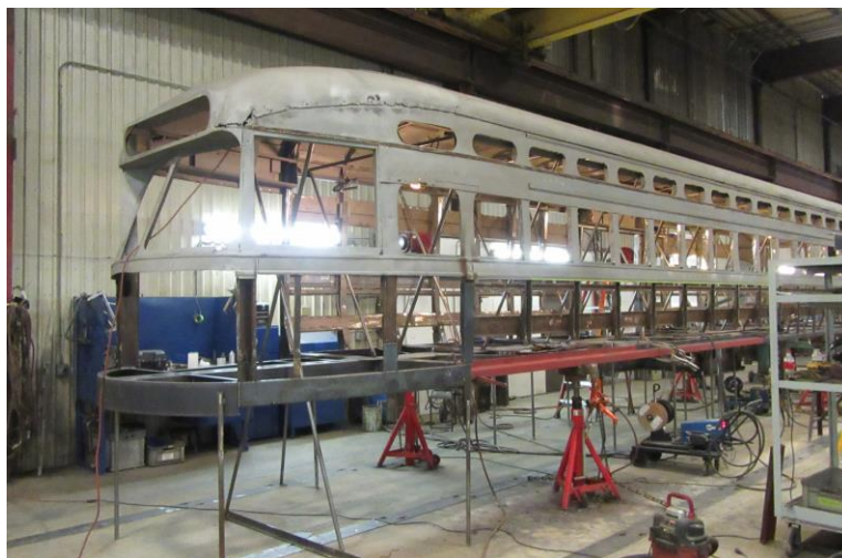
Figure 22 – Side Wall Post Bottoms Replaced
