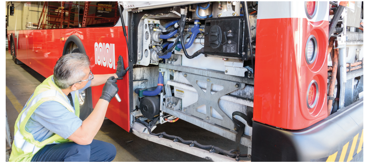
Figure 8-2 Technician Performing Preventative Maintenance
