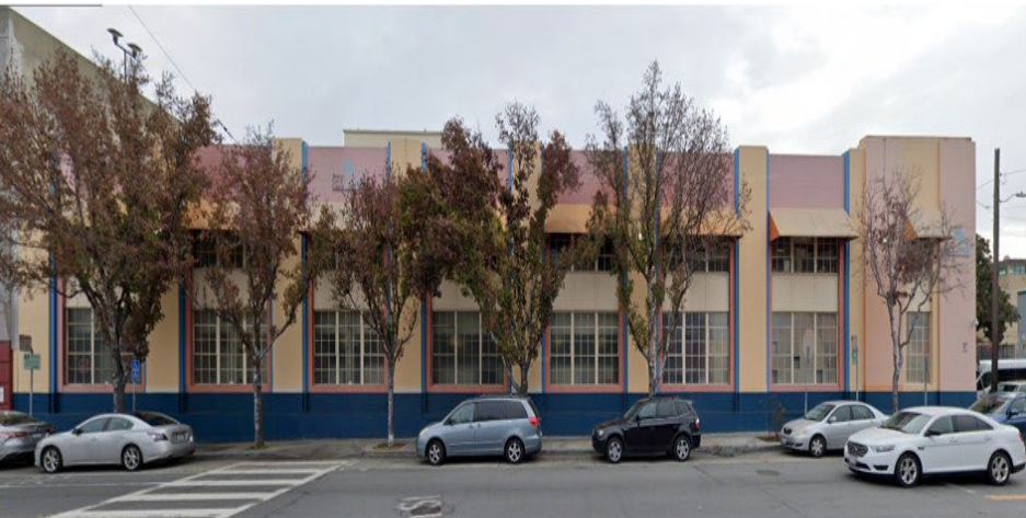
Building Elevation Facing Harrison St.
