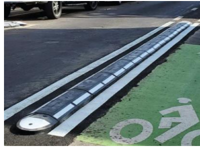
Bus Lane Curb
