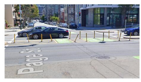
A median diverter is created by installing several traffic delineators or concrete in the middle of the intersection. Combined with turn restrictions, median diverters prevent vehicles from continuing through the intersection. Vehicles must turn right, while bicycles are allowed to ride through.
