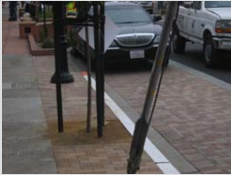
Pervious paving in the sidewalk and parking lane
