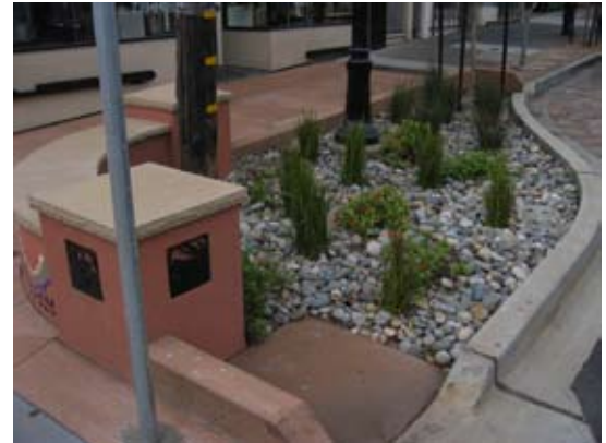
Stormwater management facilities
