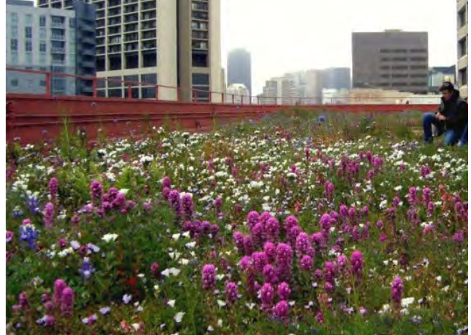
Living roof at One South Van Ness Avenue. Photo by Greenroofs.com.
