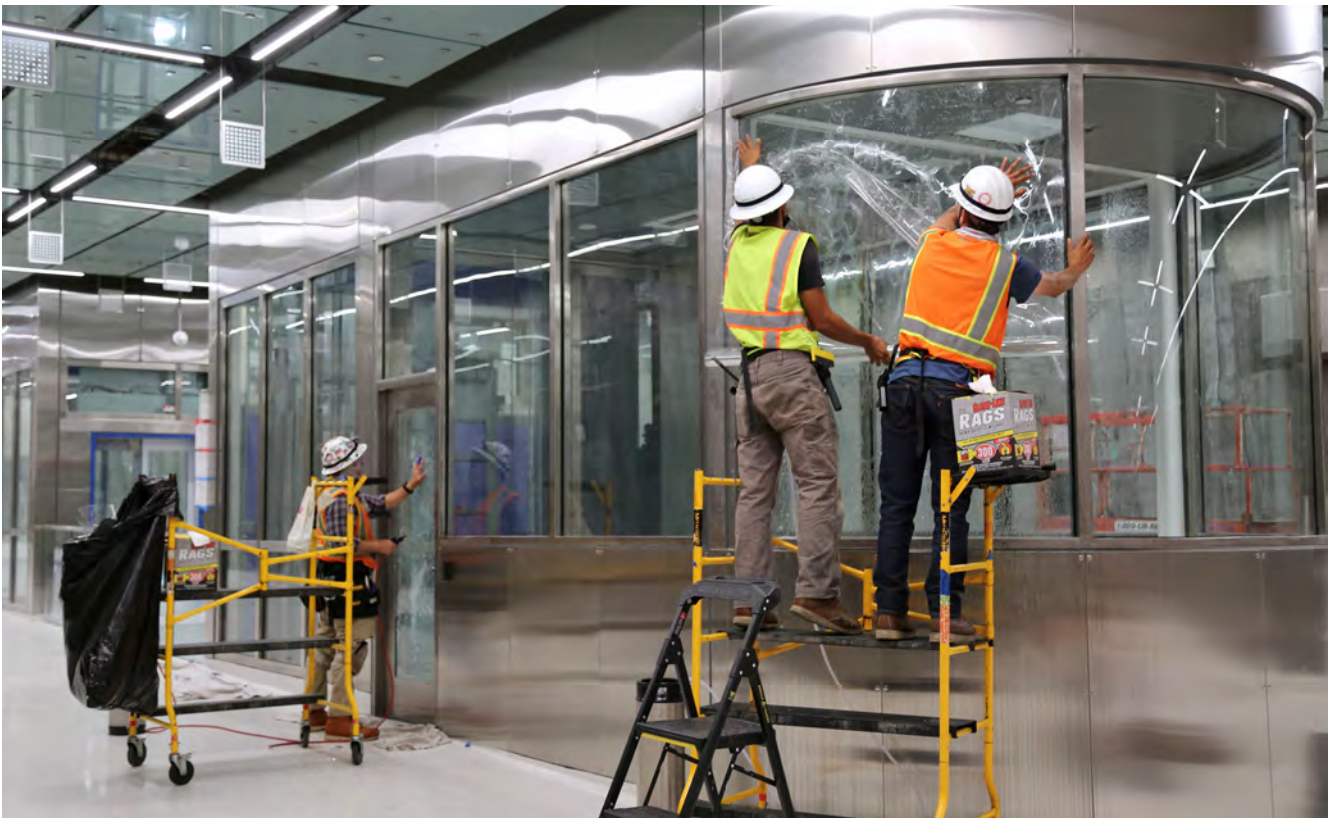
Worker installing the glass paneling for the ticketing booth at UMS
