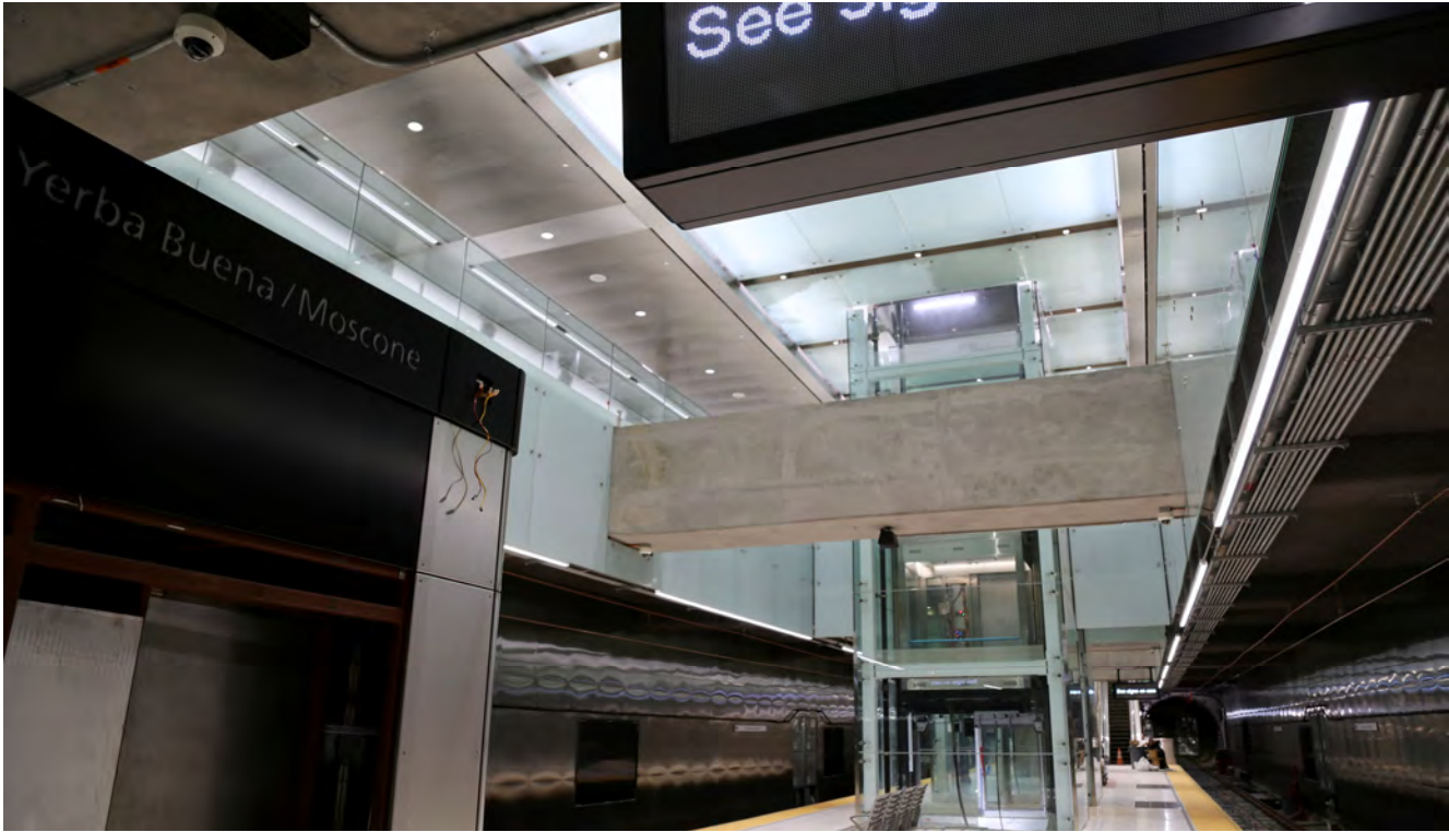
View from the platform of the elevator and seismic beams at YBM
