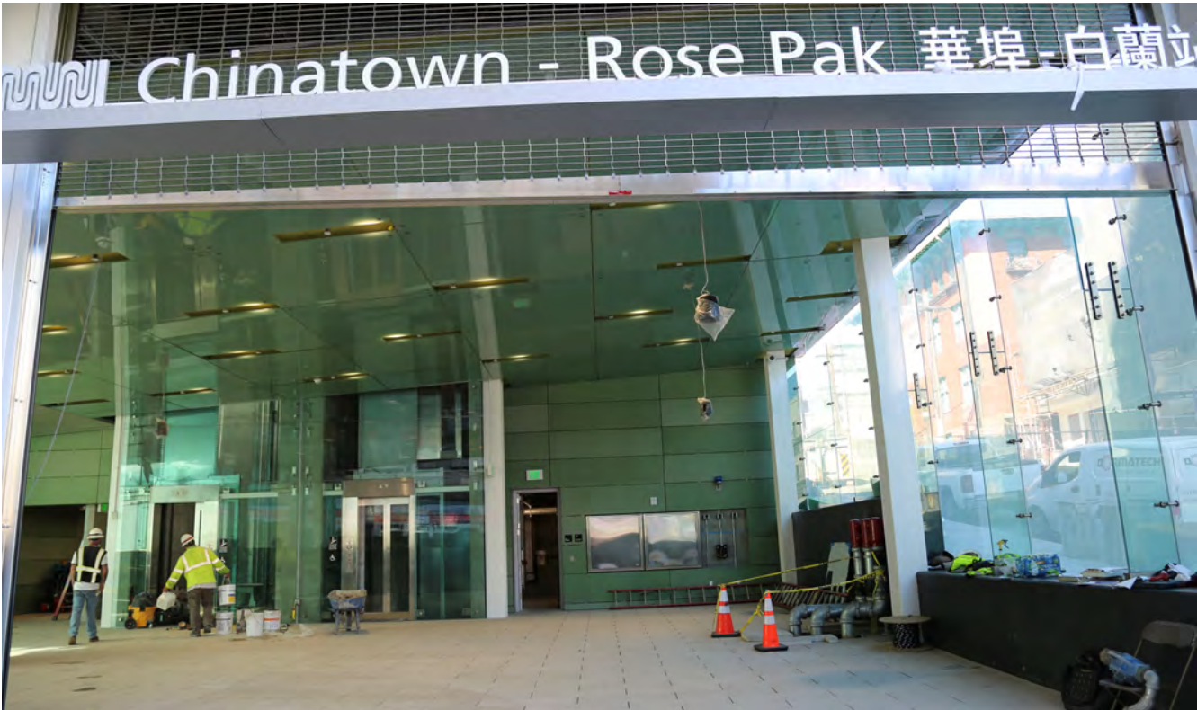
View of the entrance lobby at CTS
