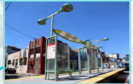
4th St. Surface Track, Systems (STS)
