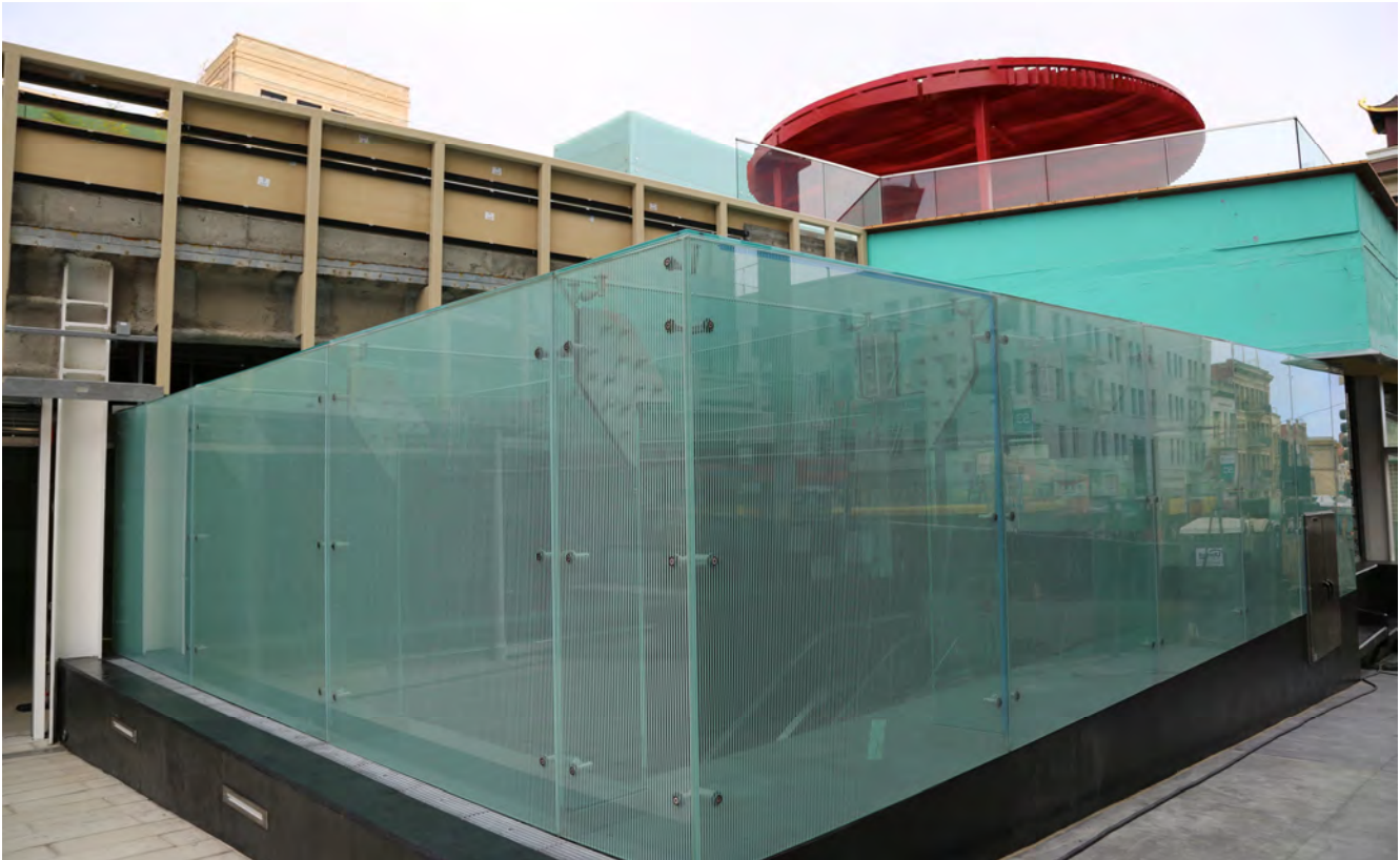
CTS Head House Glass enclosure
