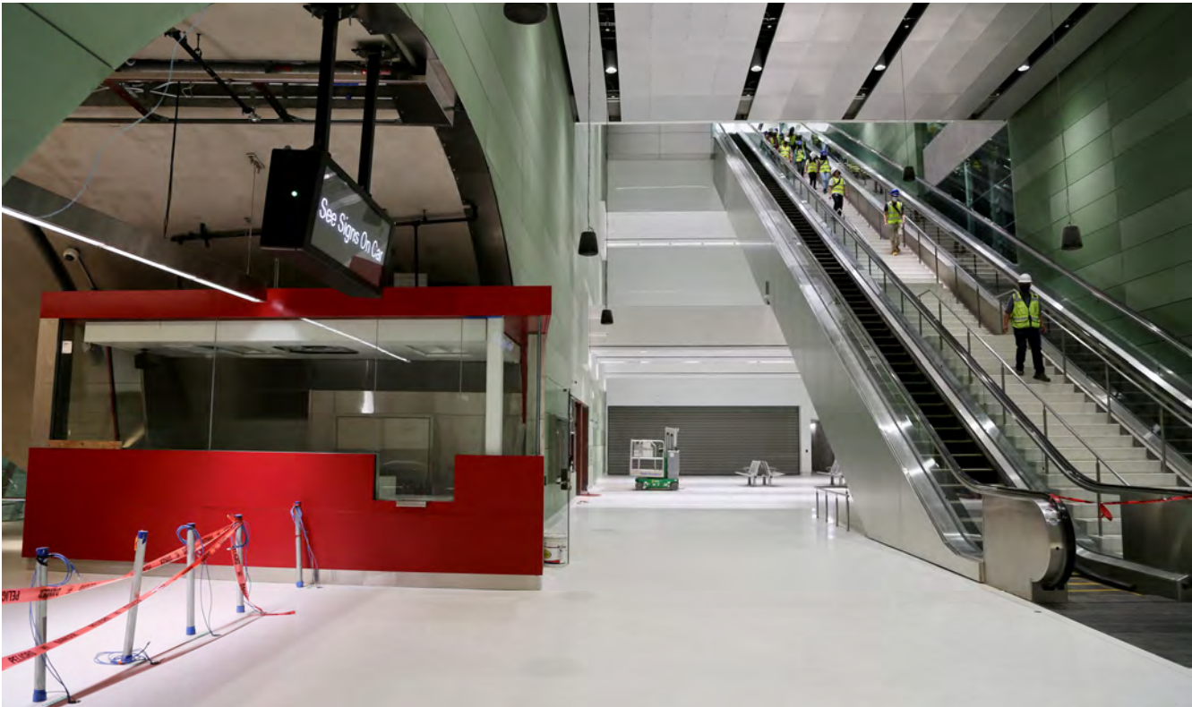
View of the ticketing lobby at CTS
