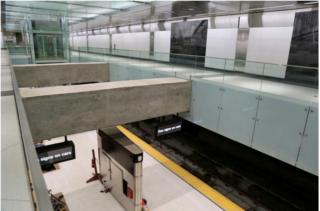
Looking down to the platform from the concourse level
