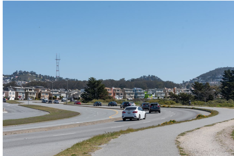
Long distances b/w crossings and gaps in signage on Lake Merced Blvd. heading eastbound towards Middlefield Dr.
