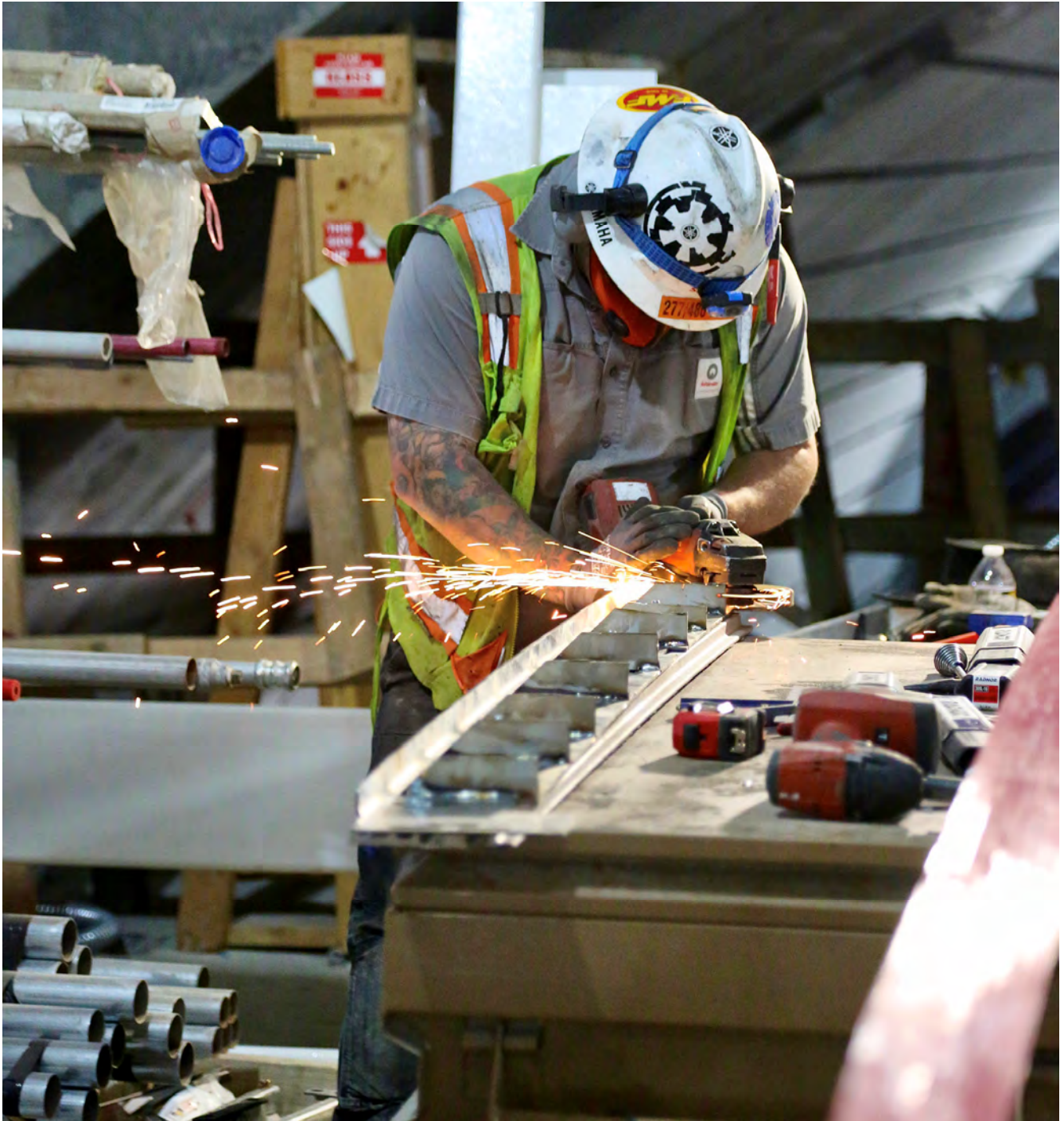
Worker cutting some material to be placed
