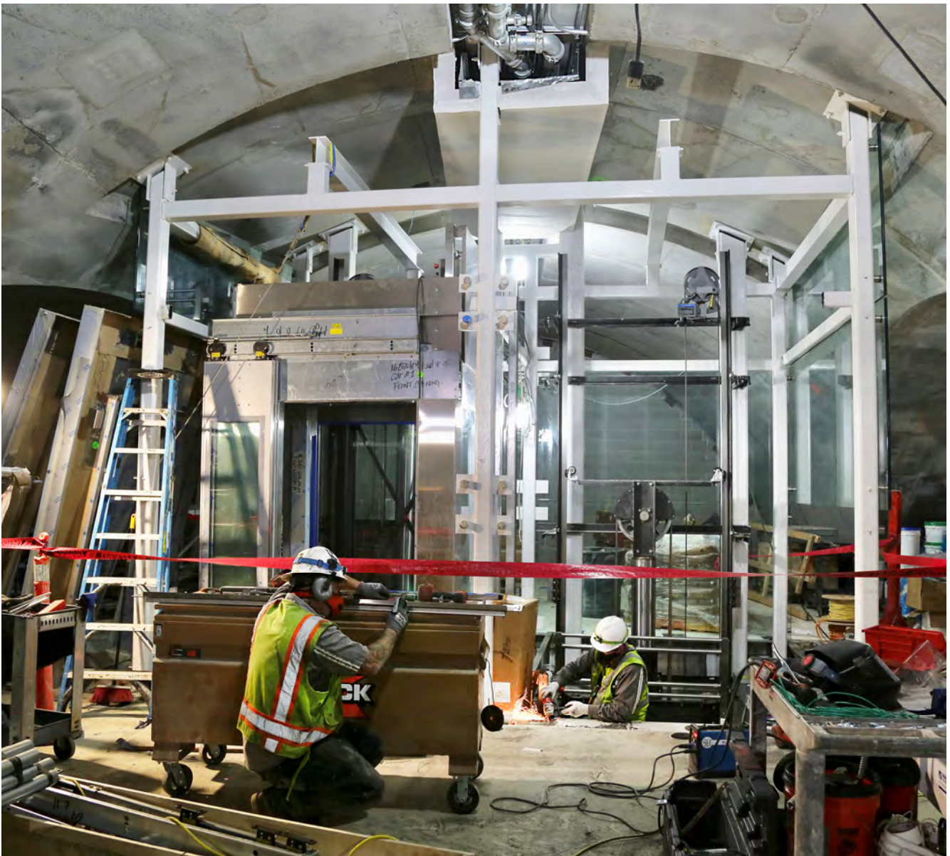
Elevators being worked on at CTS
