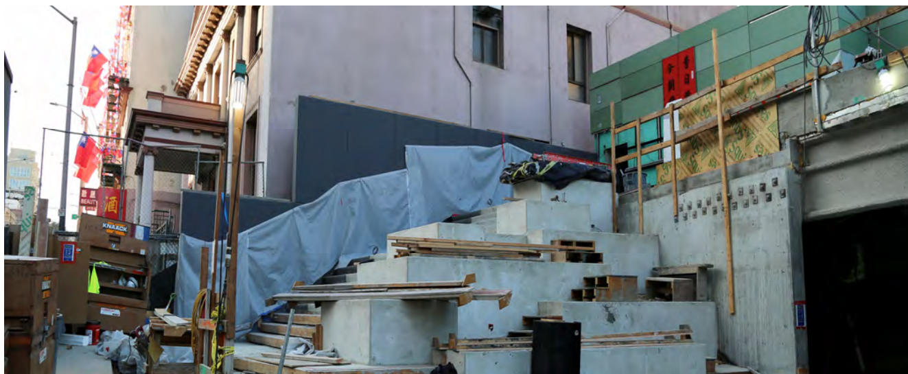
Outside progress at the Chinatown station
