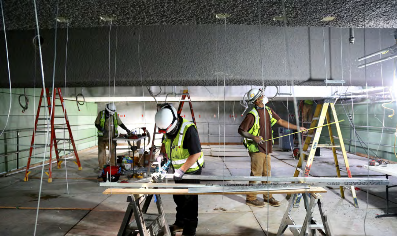
Electricians working on the ceiling wiring at CTS
