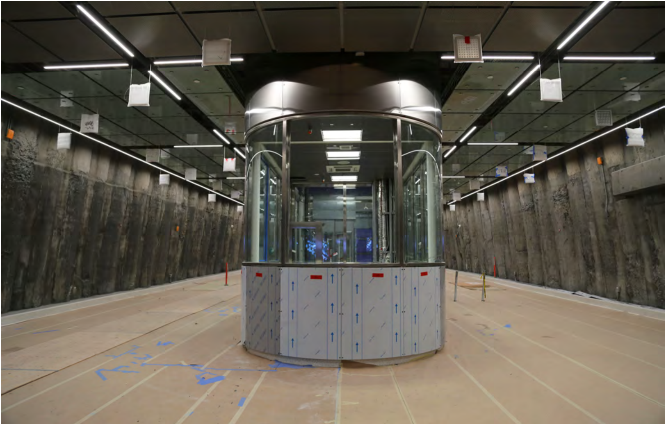
Agent booth at UMS, still being worked on
