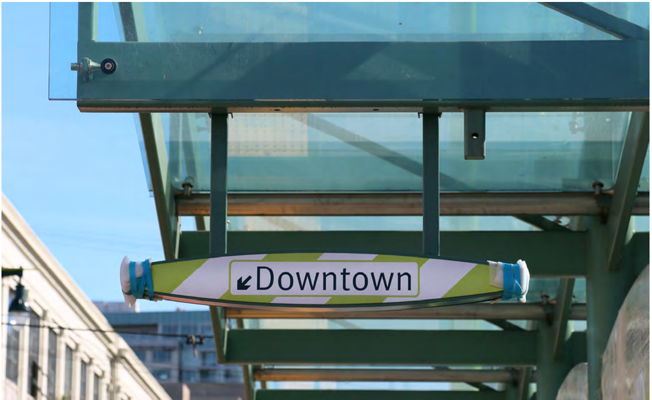
Signage on one of the surface platforms at STS
