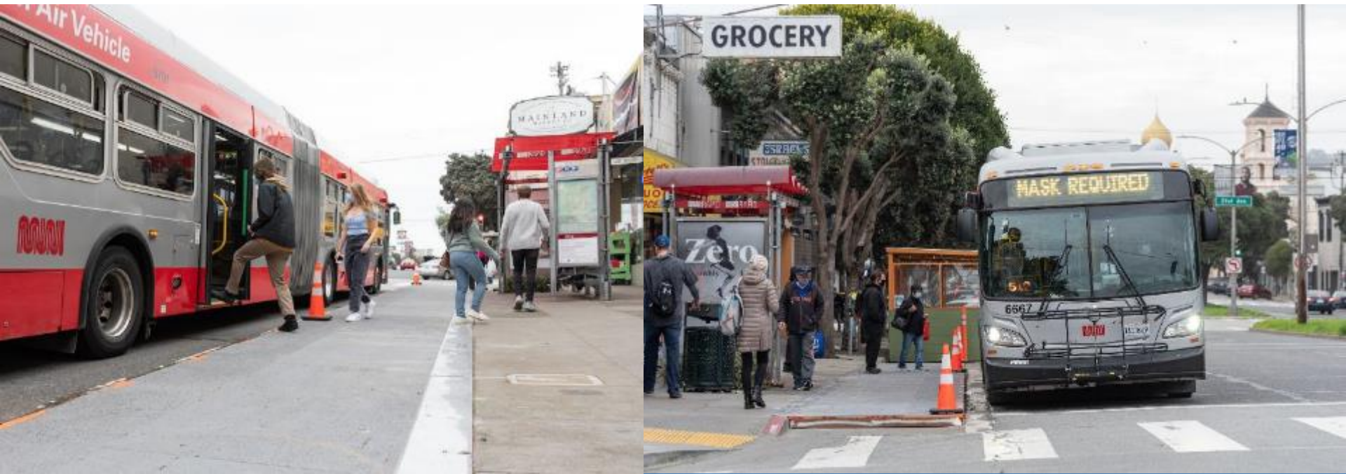
Temporary wooden bus bulbs (20 th Avenue, inbound)
