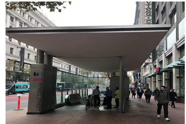
BART canopy at Powell Station on Market Street.
