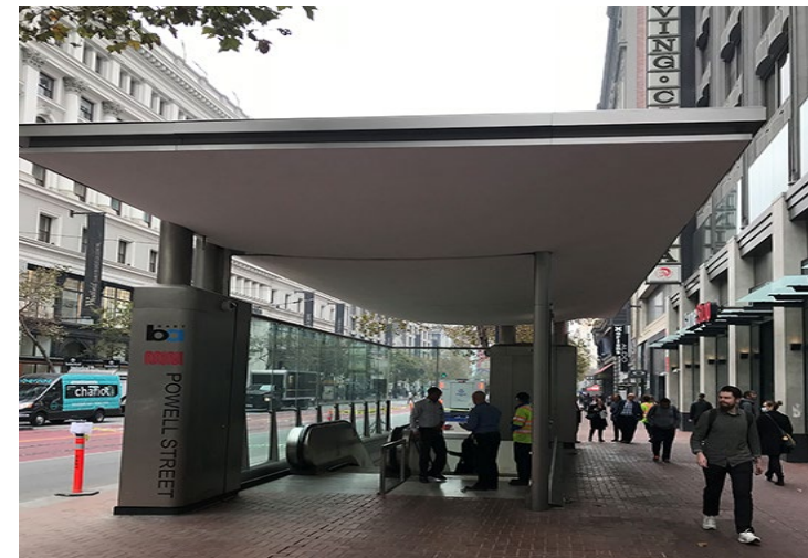
BART canopy at Powell Station on Market Street.
