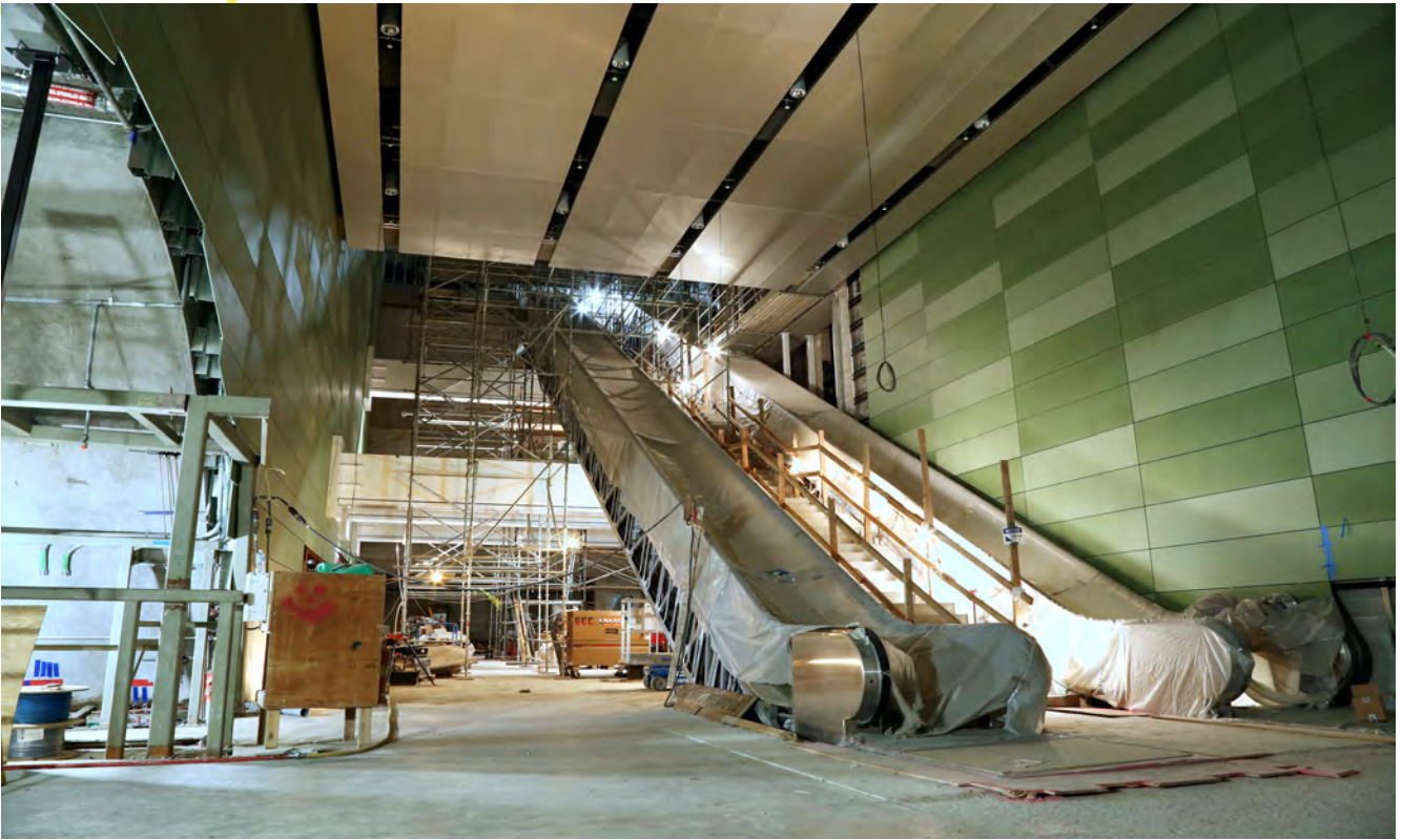
Concourse Level 1 progress at Rose Pak-Chinatown Station
