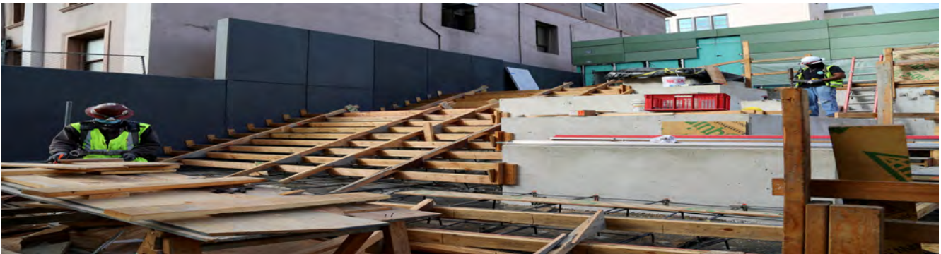
Formwork for stair at surface level of Rose Pak-Chinatown Station.
