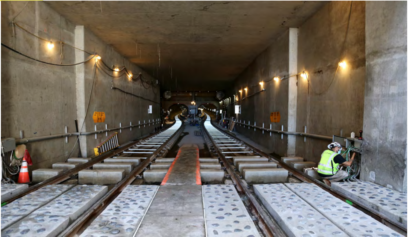
Looking into the portal entrance with worker running cables
