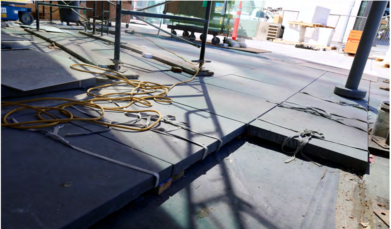
Surface level floor paneling being installed at Yerba Buena Station
