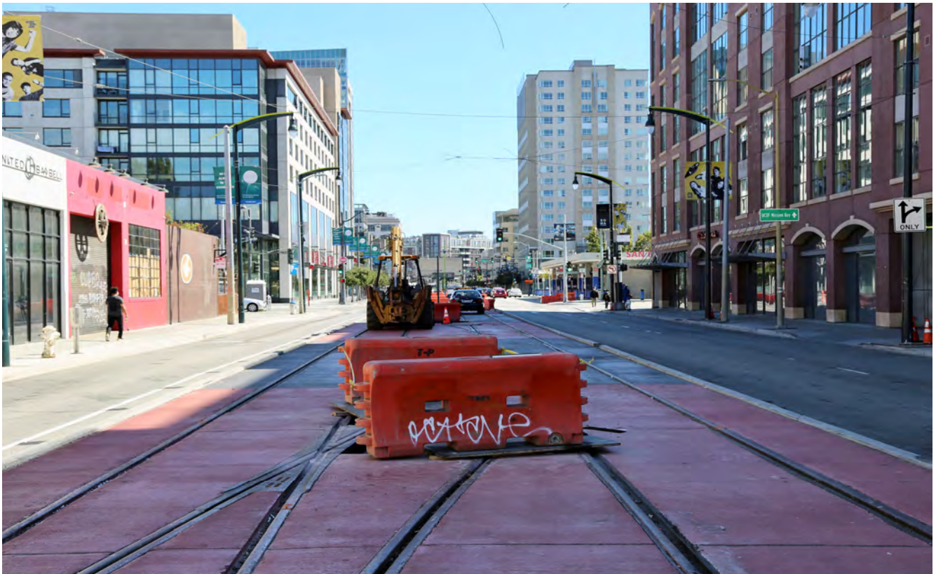
View of surface station between Bluxome St and Townsend St
