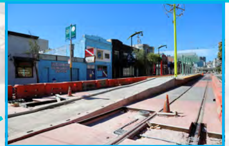
4th St. Surface Track, Systems (STS)
