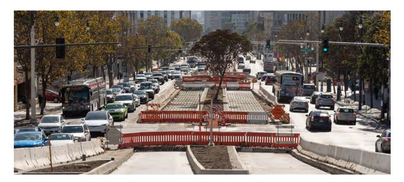
Residents of Van Ness may have noticed switches in traffic patterns in September and November. This switch allowed crews to create a work zone in the middle of the roadway, and begin constructing the Bus Rapid Transit (BRT) system.
