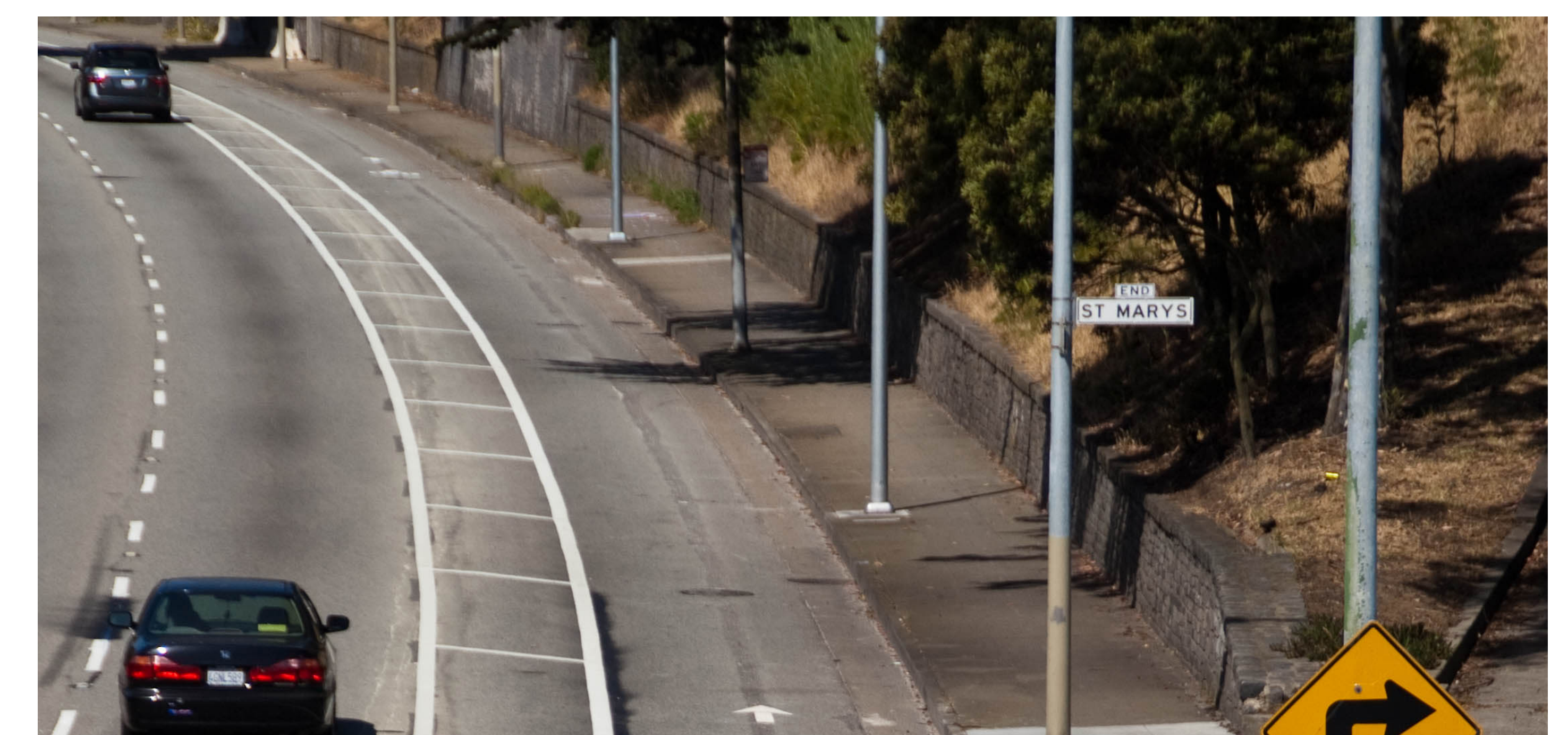
Existing Painted Buffer
