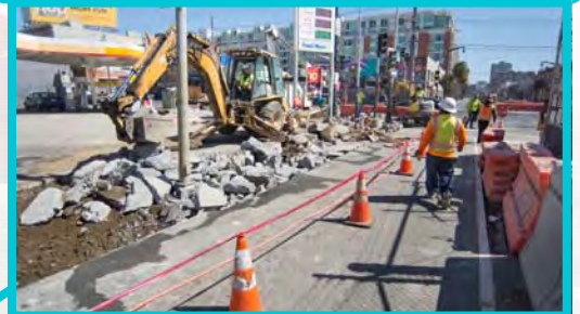
4th St. Surface Track, Systems (STS)
