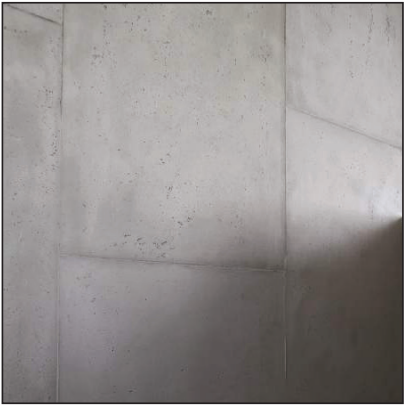
Poured in Place Concrete
