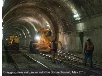
Dragging new rail pieces into the Sunset Tunnel, May 2015.
