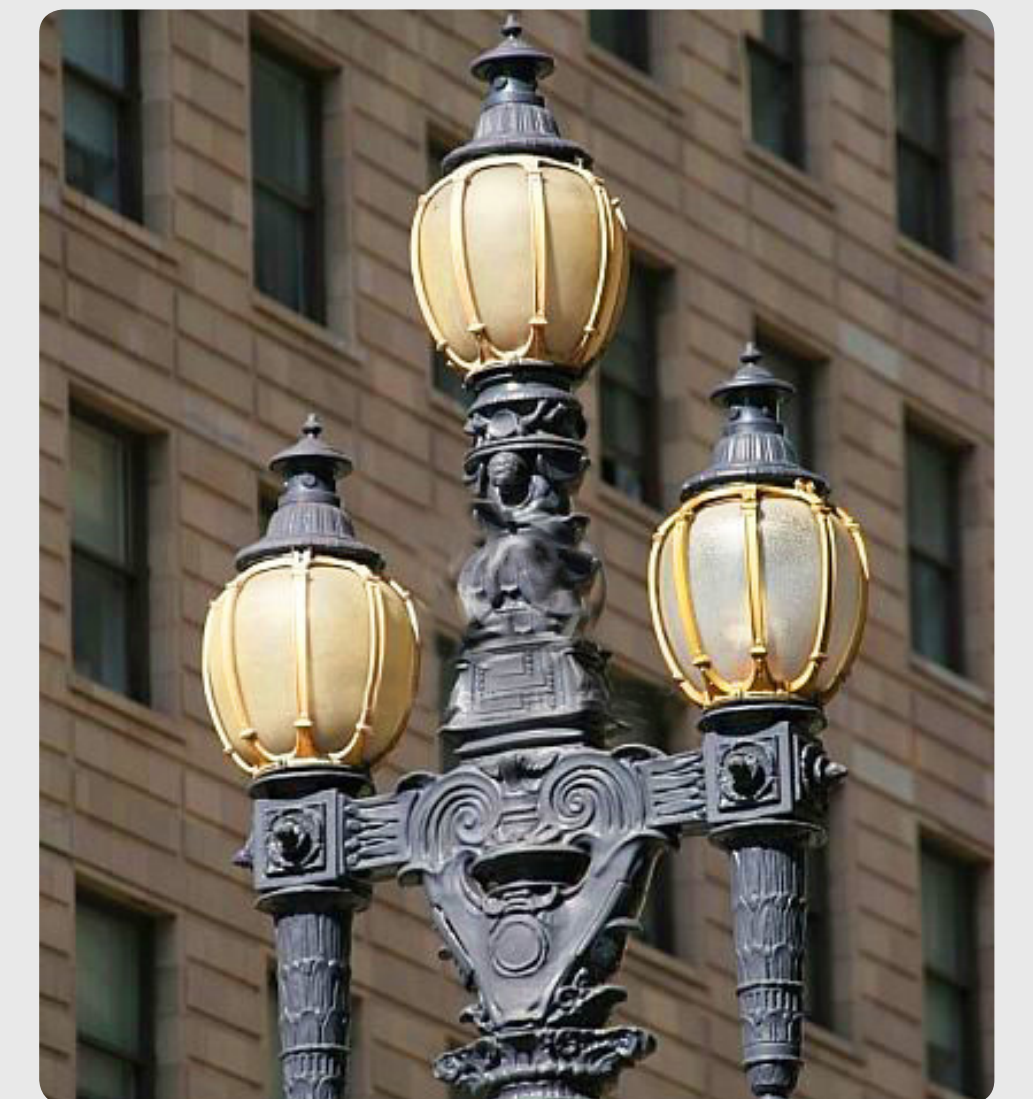
Restore "Path of Gold" Light Fixtures LED conversion & powdercoat touch-up
