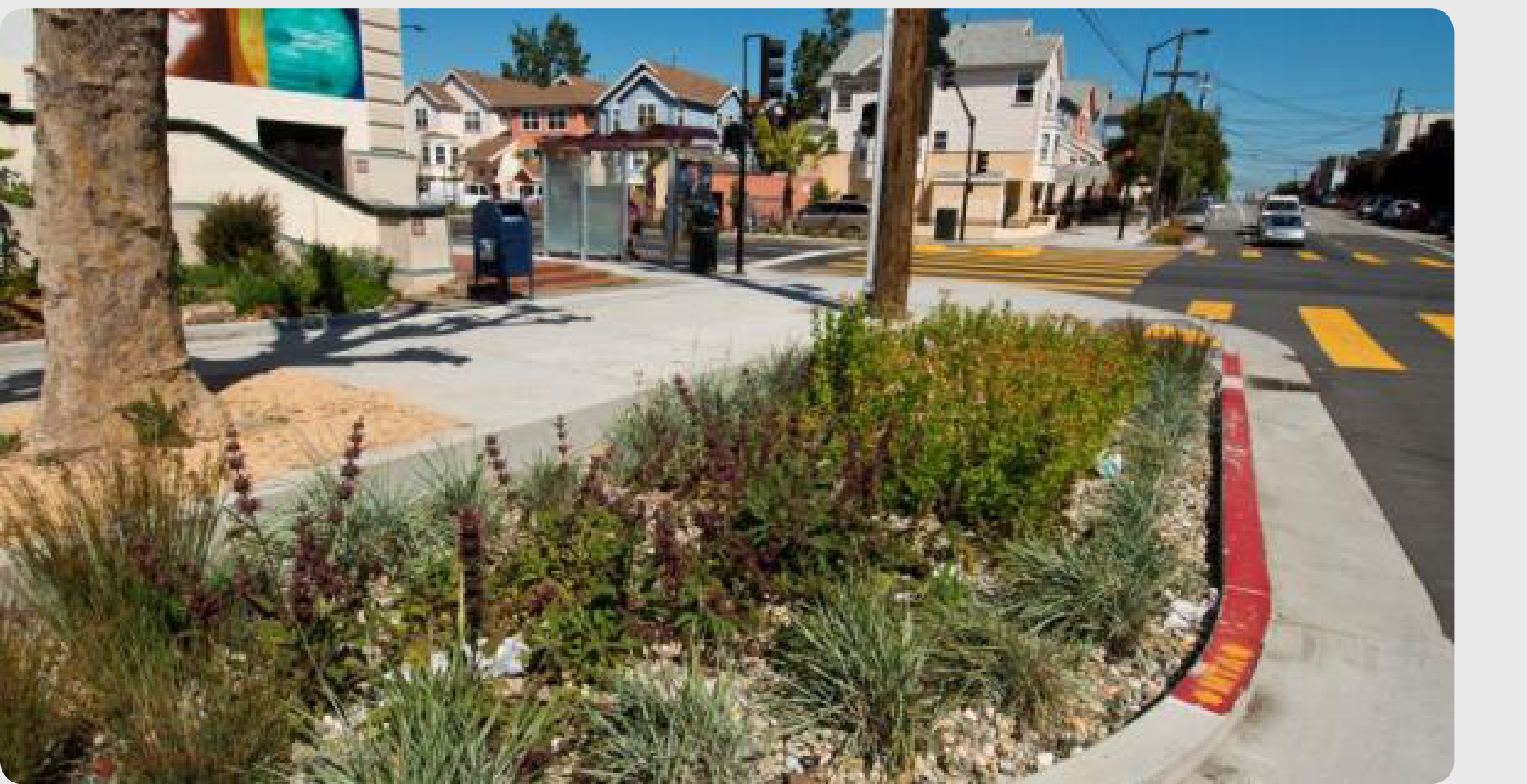
Green Infrastructure at Bulb-outs Further analysis is required to determine feasibility and potential locations
