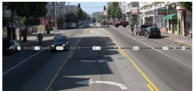
Road Diet: When the number of vehicle lanes or effective width of a road is reduced in order to achieve systemic improvements, turning movements and bicycle lanes, often related to safety.
