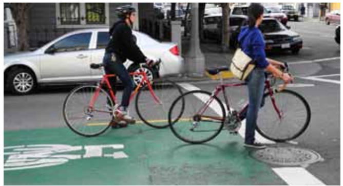
Green Bicycle Boxes: On-street markings at signalized intersections that provide space to queue and advance in front of vehicle traffic with the use of an advanced stop bar.
