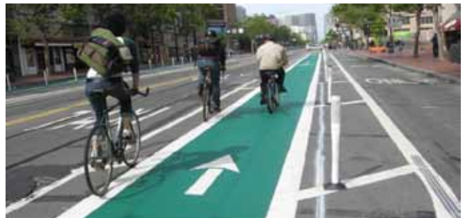
Cycle Track: An exclusive bicycle facility within the roadway that is physically separated from motor vehicle traffic through the use of bollards, car parking, barriers, or boulevards, and may have one-way or two-way operations.
