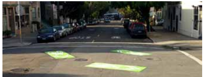
Sharrows/Painted Sharrows: On-street markings placed in the travel lane to indicate to motorists and riders that the lane is shared with people on bicycles, and that both may use the full lane.
