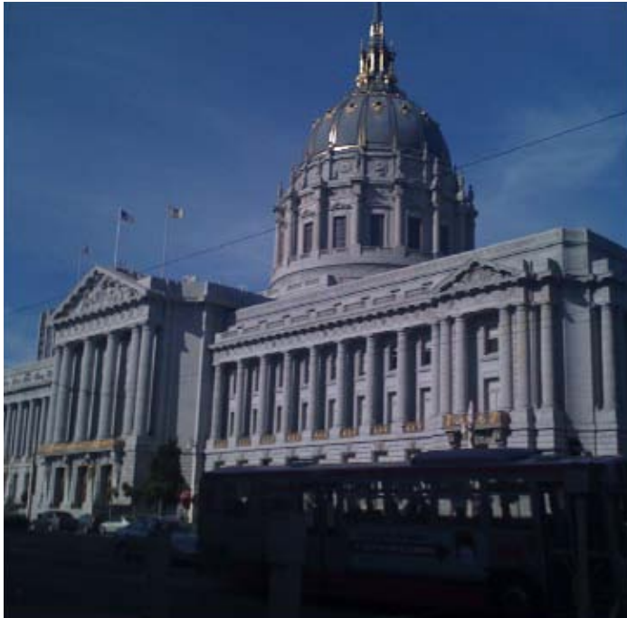
Image: Picture of City Hall on the Van Ness Street side with articulated trolley bus in front.
