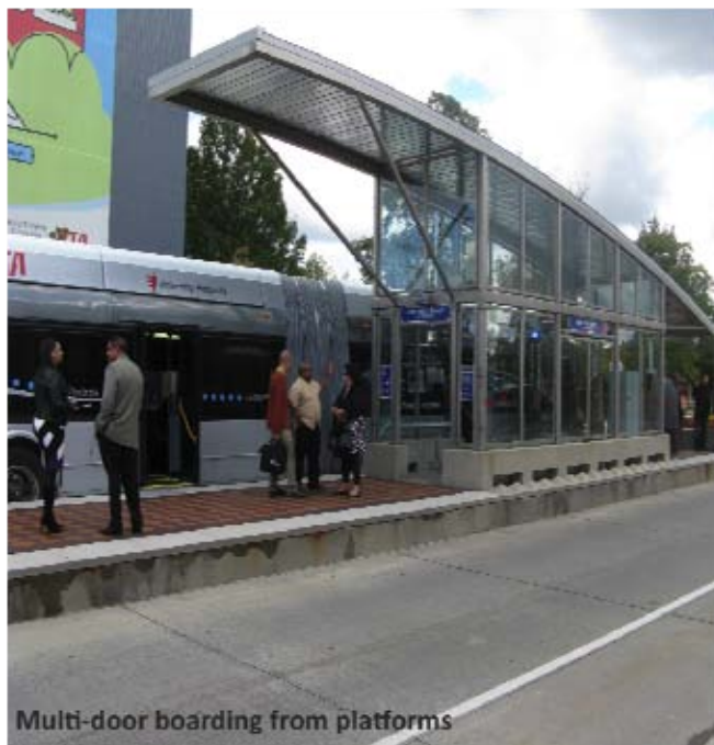
Image: photograph shows a light rail vehicle loading passengers from a platform that has a glass covered exit for passengers.
