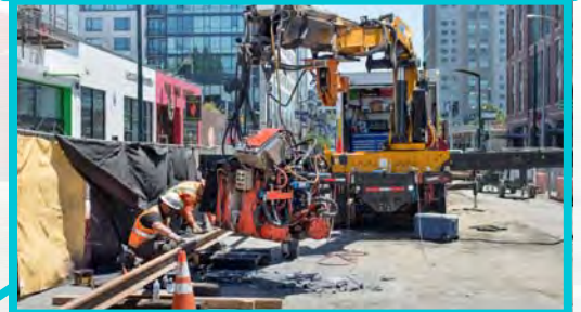
4th St. Surface Track, Systems (STS)
