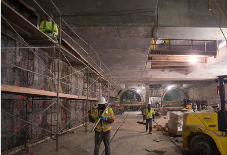
1 Steel reinforcing and shotcrete are applied to build exterior walls
