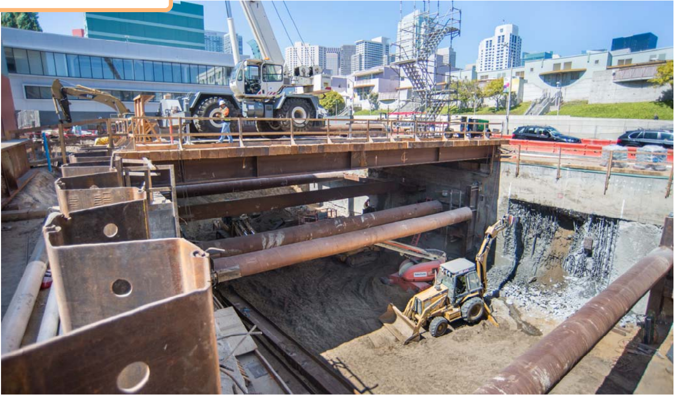
The partially-excavated headhouse structure, at 4th and Folsom.
