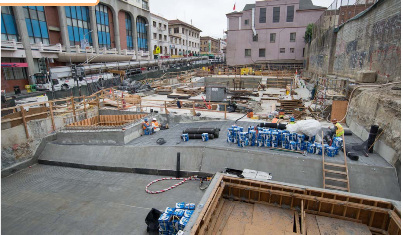
With concrete poured, workers will begin waterproofing the surface and backfill.
