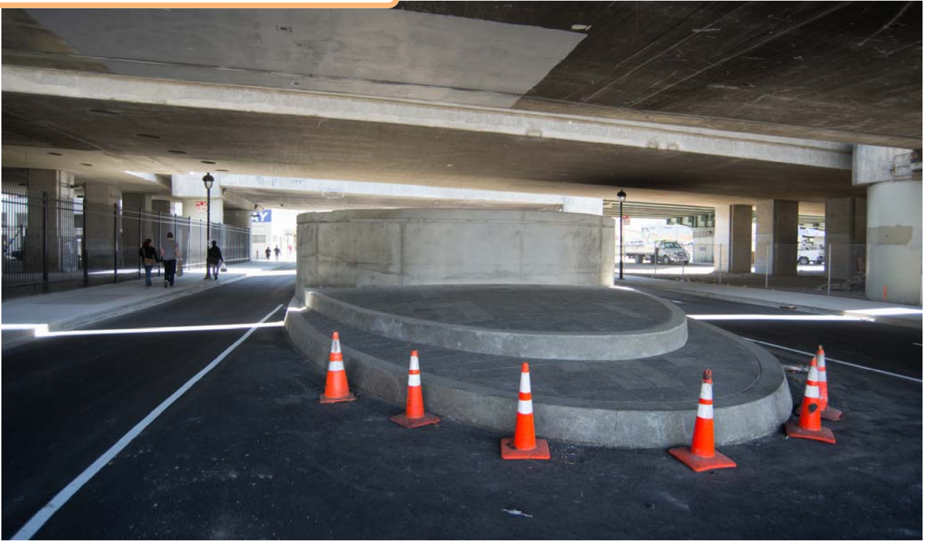
The approach and curb of the tunnel portal can be seen here, under the Interstate 80 overpass.
