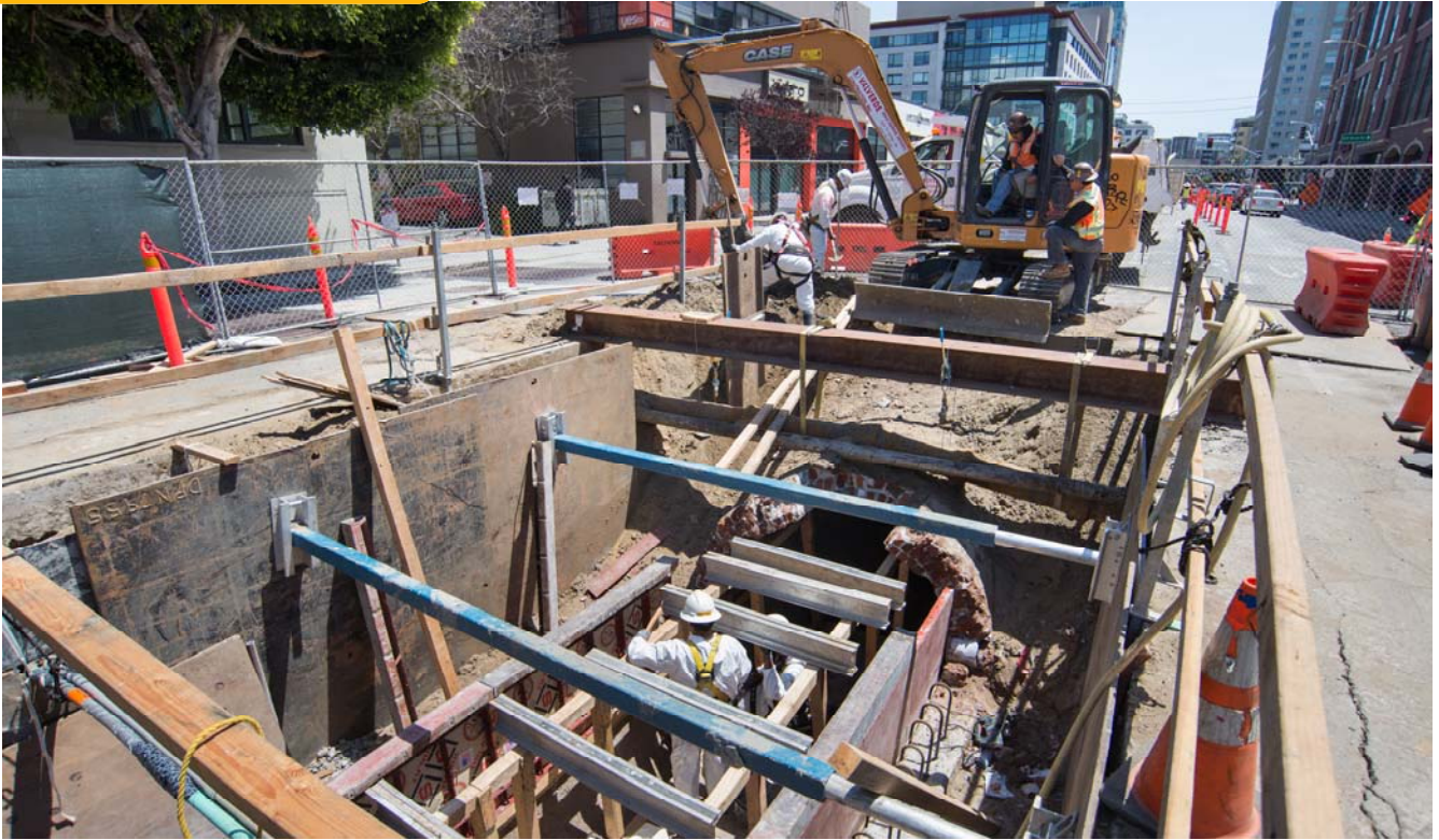
Workers install rebar and forms ahead of pouring concrete for the reconstructed 78-inch sewer just south of Brannan on 4th.
