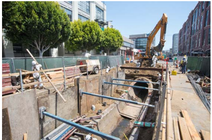
This century-old brick sewer is getting a new lease on life with a reinforced concrete roof, on 4th Street south of Brannan.
