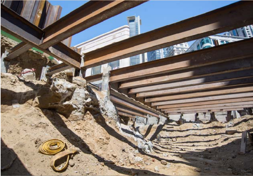
1 Major structural roof elements are installed and reinforced
