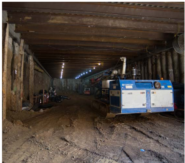
3 Soil improvement is ongoing outside the walls of the already-covered portion
