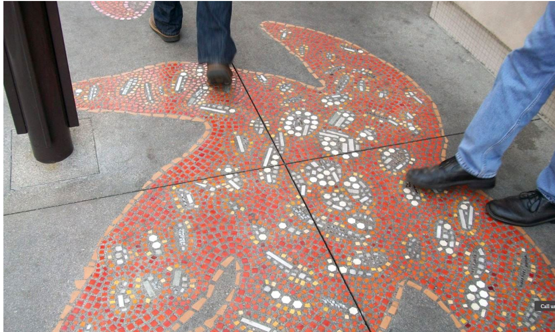
Example of decorative sidewalk with glass aggregate
